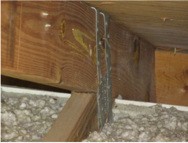
Double wraps roof to wall Attachment
