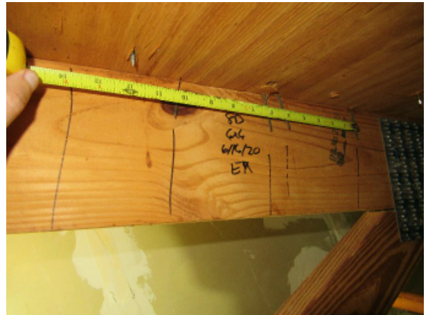
8d nails 6x6 Roof Deck Attachment
