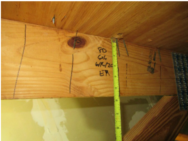
8d nails 6x6 Roof Deck Attachment
