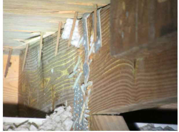
Double wraps roof to wall Attachment
