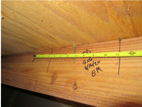
8d nails 6x6 Roof Deck Attachment
