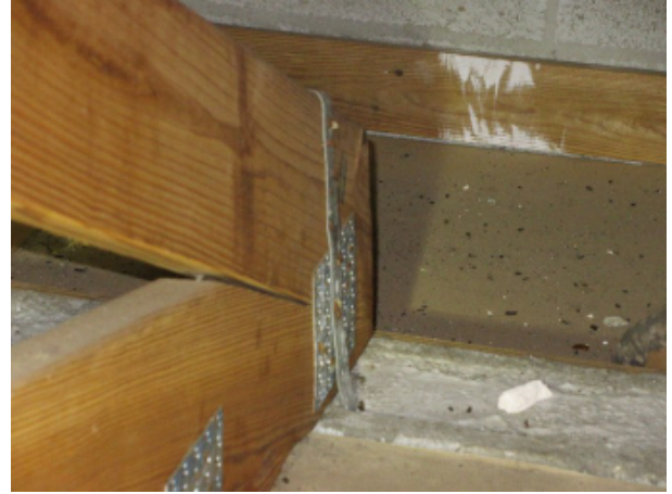
Single wrap Roof To Wall Attachment
