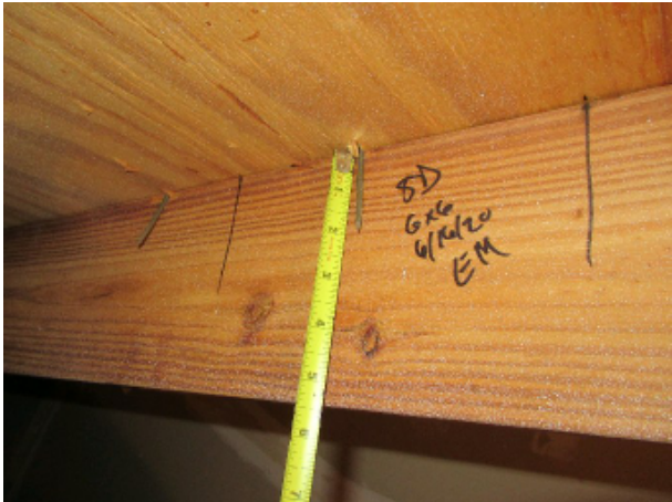
8d nails 6x6 Roof Deck Attachment
