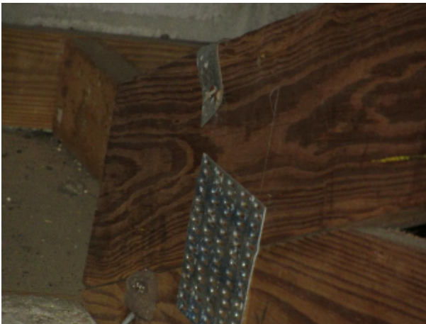
Single wrap Roof To Wall Attachment
