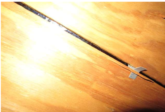
SWR installed under the tile
