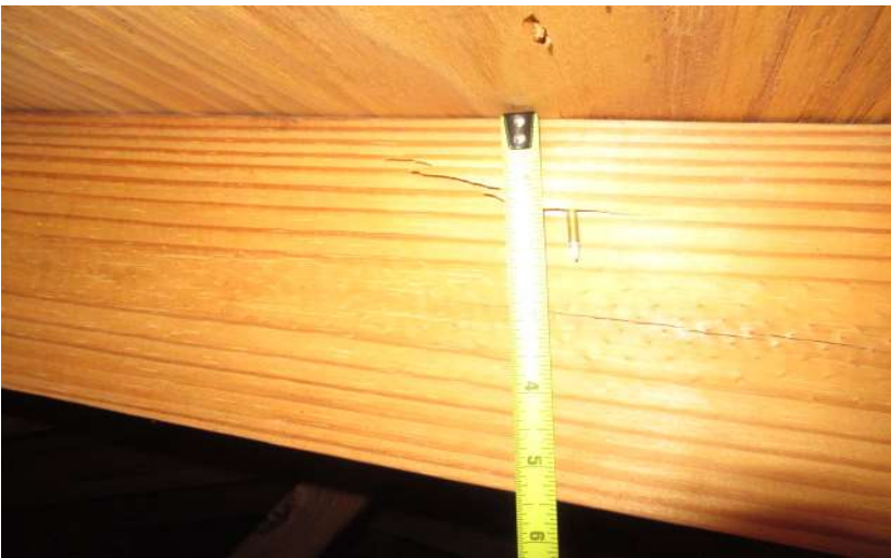
8d nails verified
