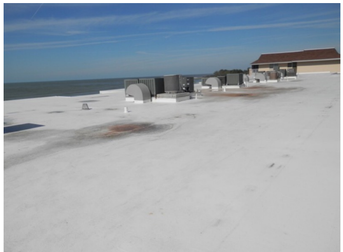
Reinforced concrete w/ membrane
