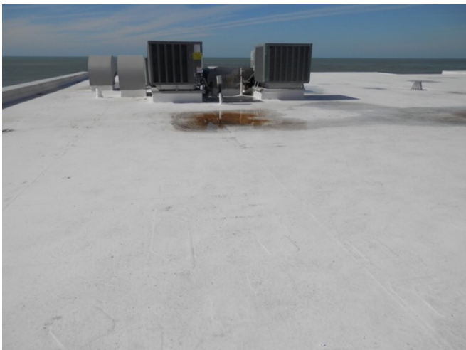
Reinforced concrete w/ membrane
