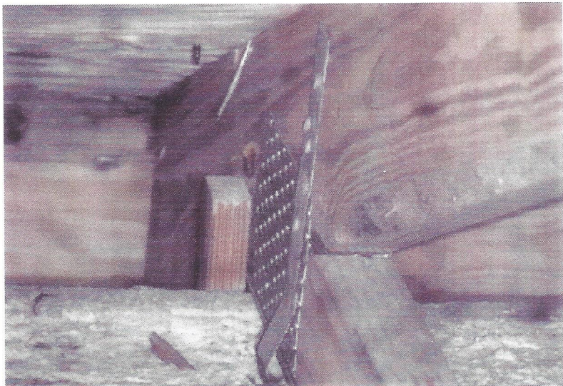
Single strap (clip) with at least 3 nails into the truss
