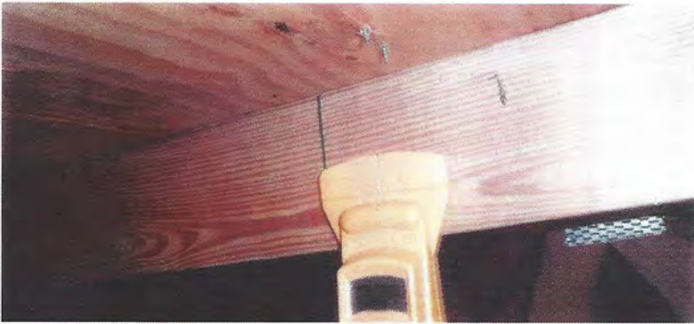
Nail location verified
