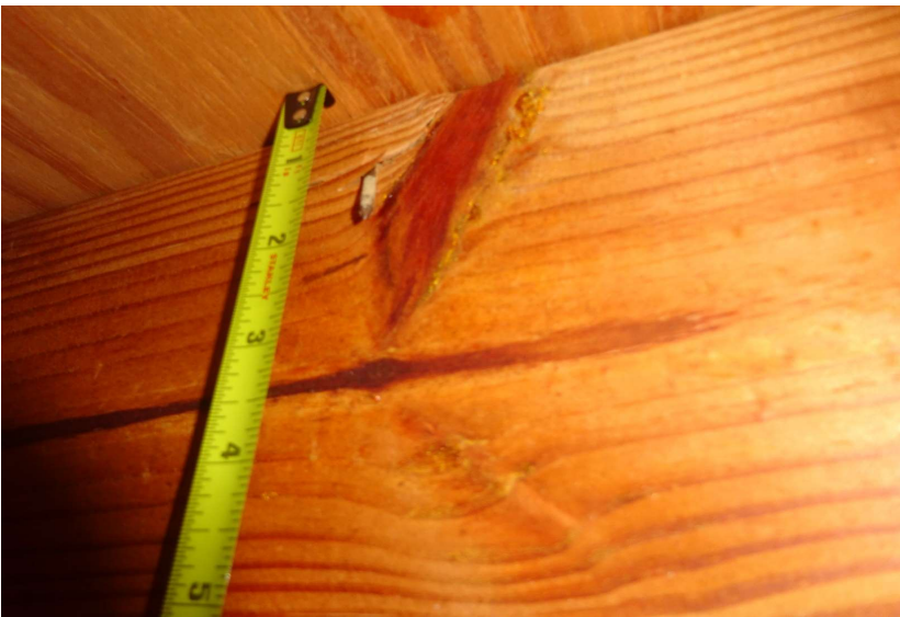
8d nails verified
