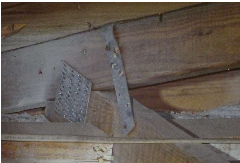
and at least 1 nail on the wrapped side
