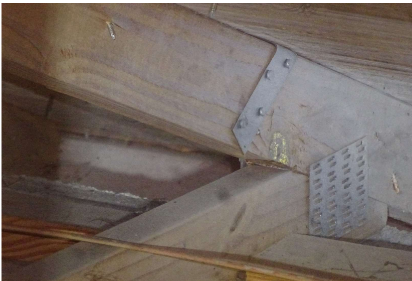
Single wrap with at least 2 nails on the embedded side and at least 1 nail on the wrapped side
