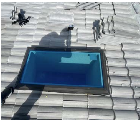
Impact Rated Skylight(s)
