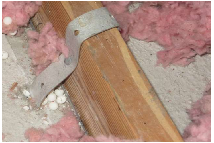
Strap with 2 nails into the truss
