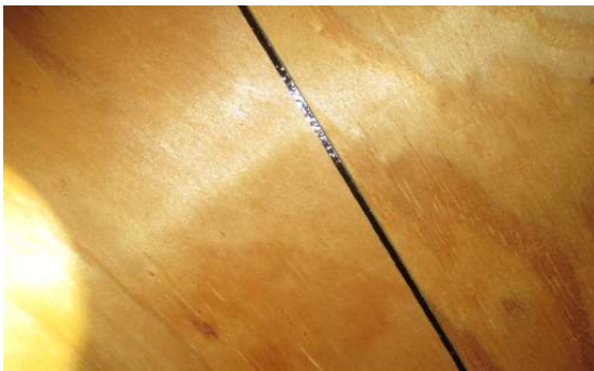
SWR installed under the shingles
