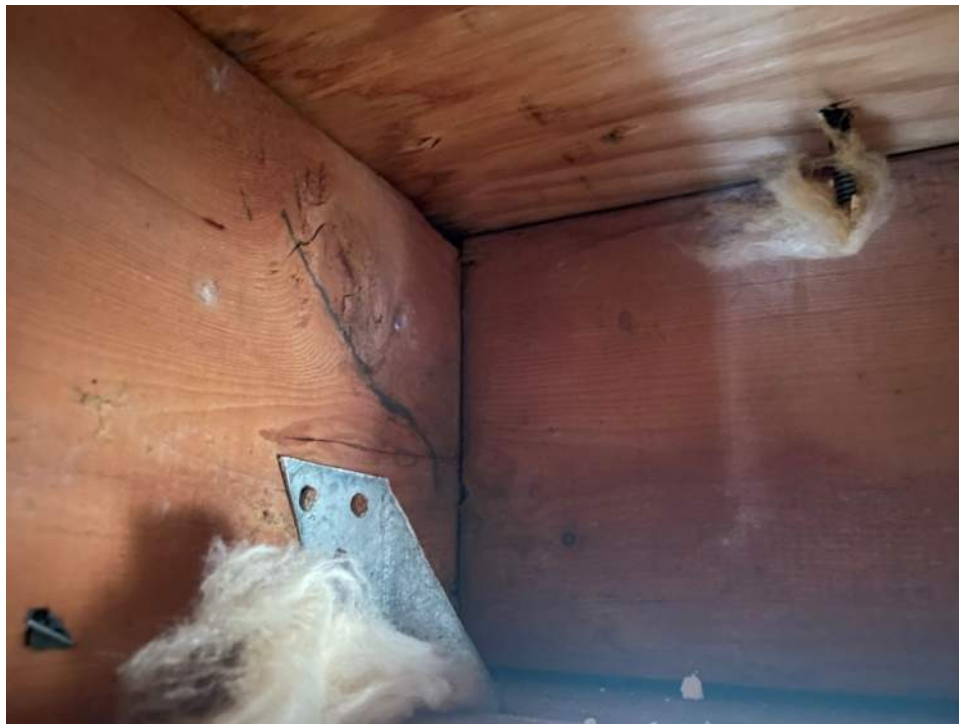
Figure 4 - Roof to Wall Attachment – Clips
