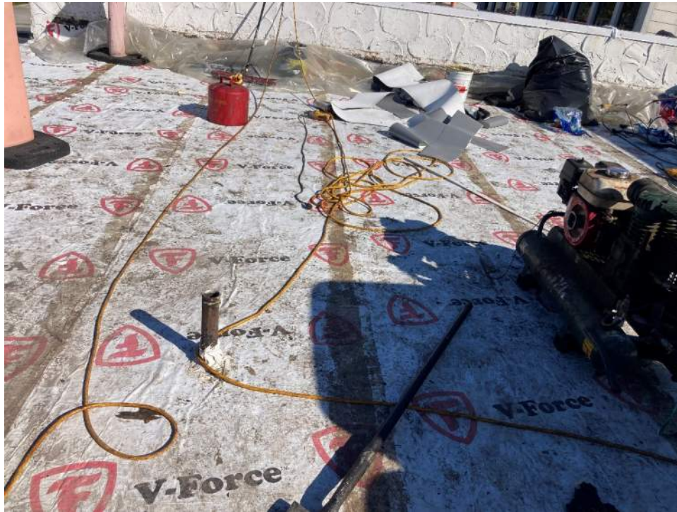
Figure 5 – Secondary Water Resistance - Yes
