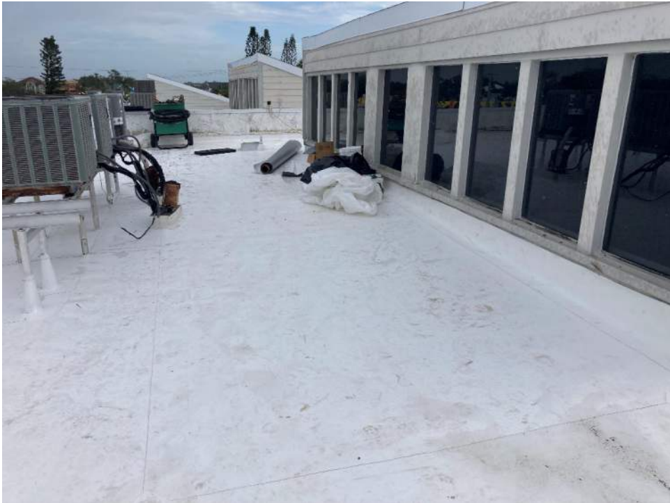
Figure 2 – TPO Roofing System
