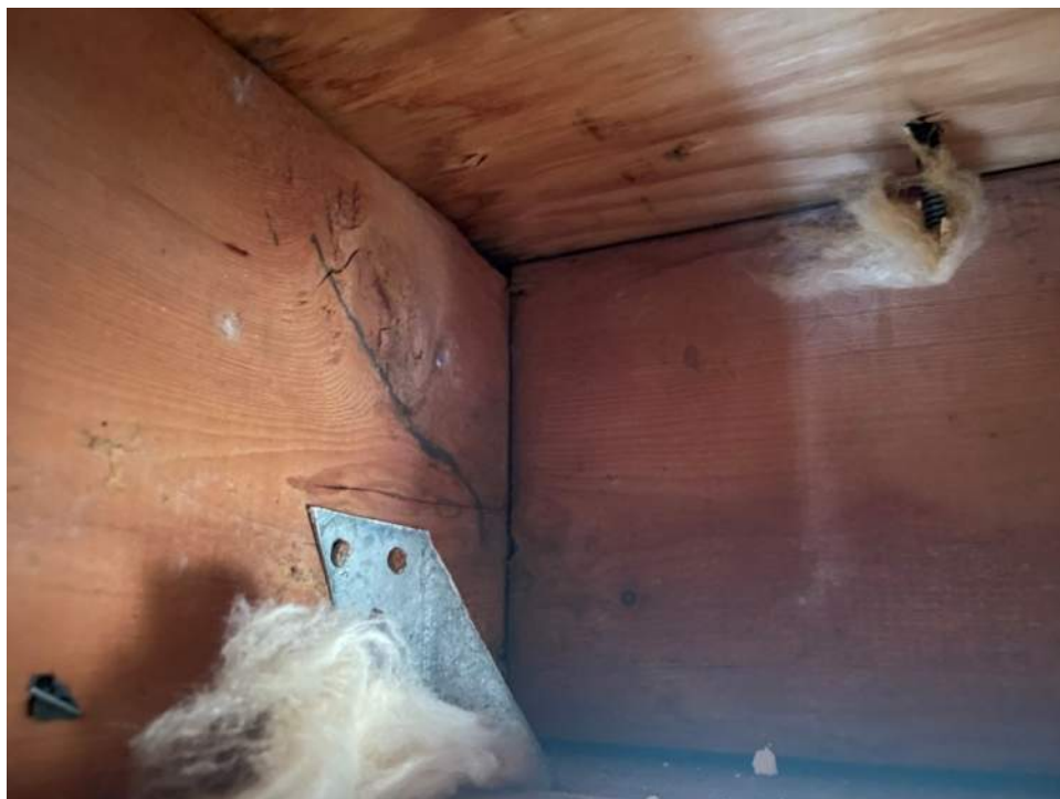
Figure 4 - Roof to Wall Attachment – Clips
