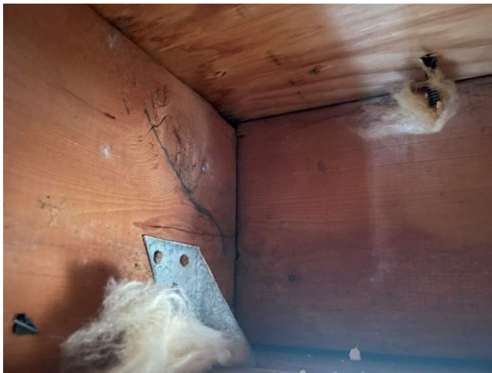
Figure 4 - Roof to Wall Attachment – Clips
