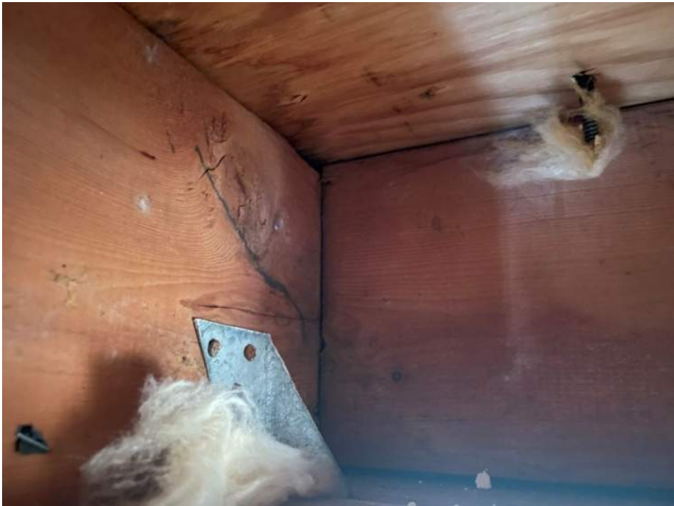
Figure 4 - Roof to Wall Attachment – Clips
