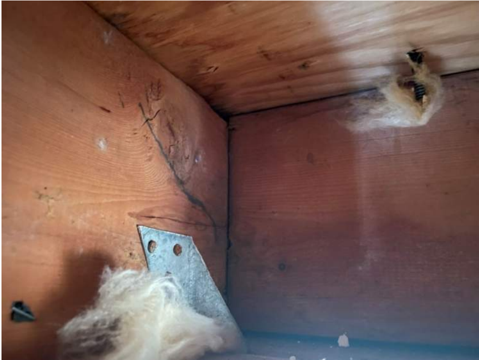
Figure 4 - Roof to Wall Attachment – Clips
