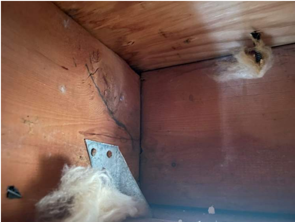
Figure 4 - Roof to Wall Attachment – Clips
