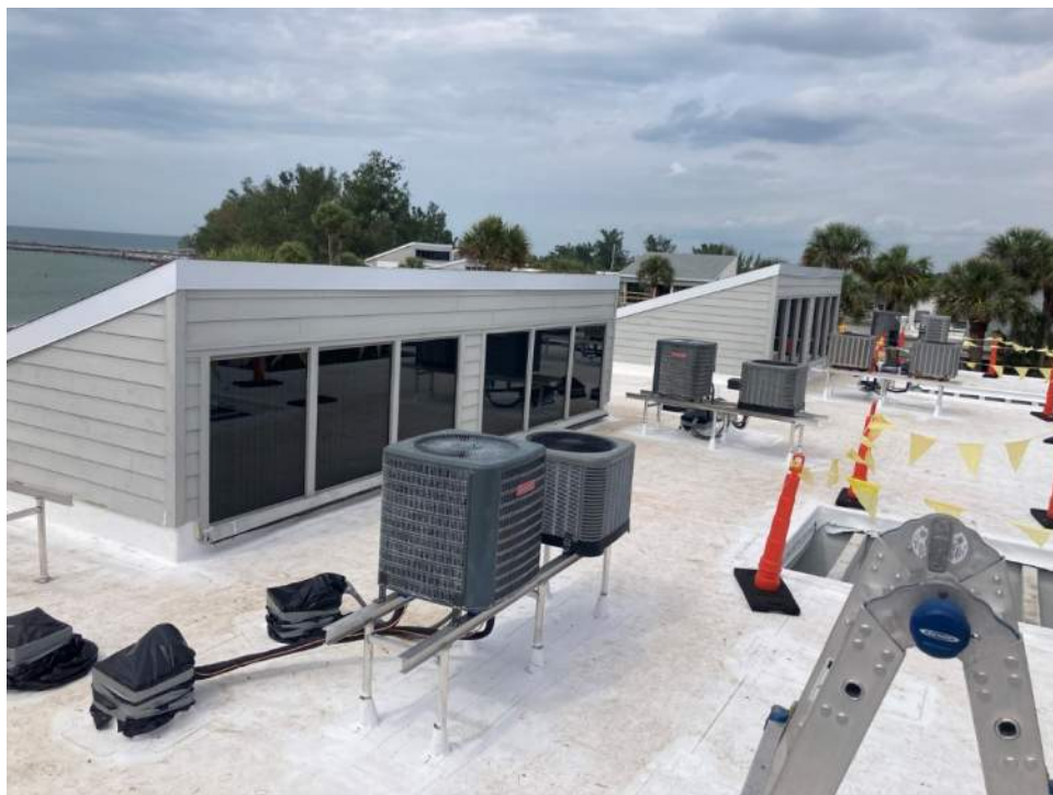
Figure 2 – TPO Roofing System
