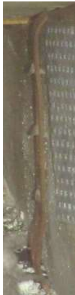
Single strap with at least 3 nails into the truss
