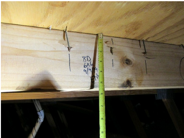
8d nails 6x6 Roof Deck Attachment
