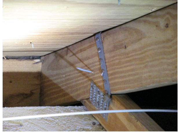
Single wrap Roof To Wall Attachment
