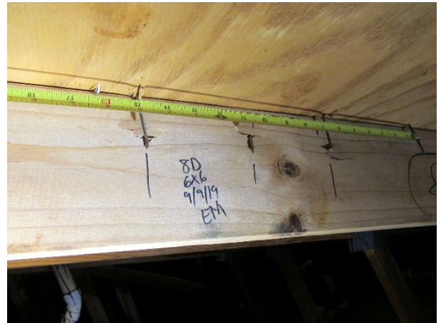
8d nails 6x6 Roof Deck Attachment
