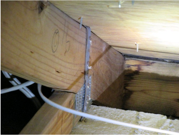
Single wrap Roof To Wall Attachment
