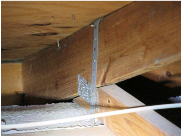
Clips Roof To Wall Attachment
