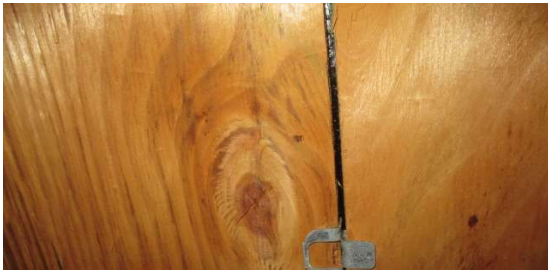
SWR installed under the shingles
