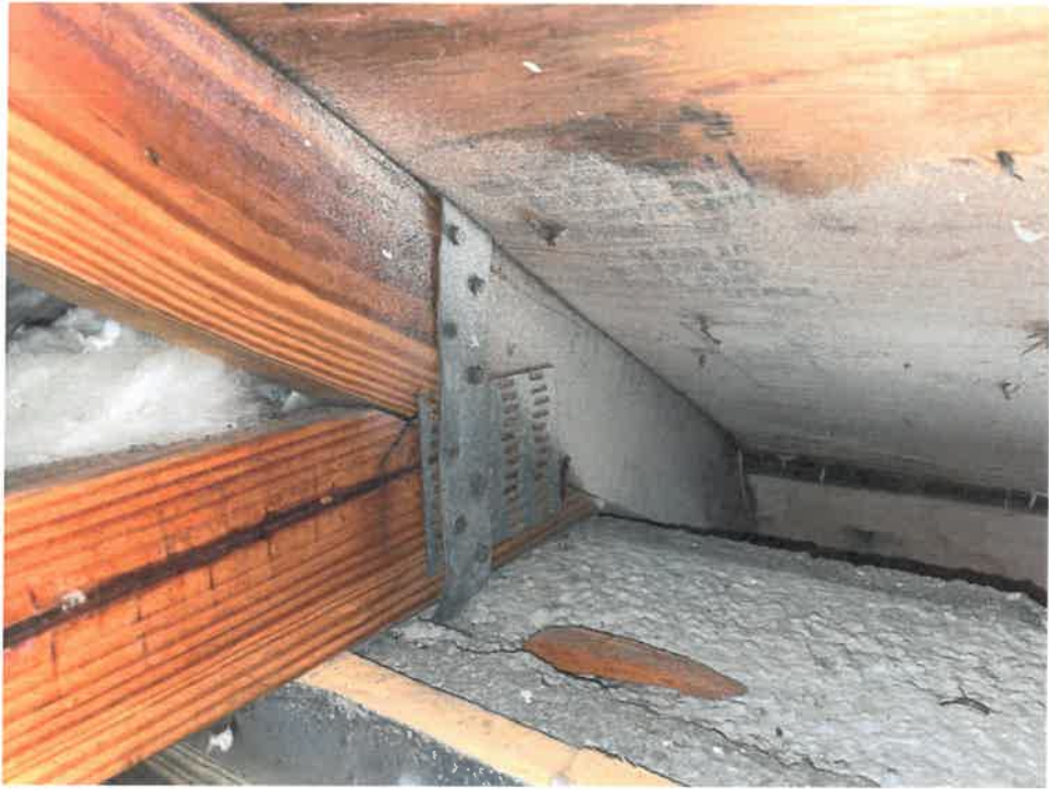
Figure 5 – Roof to Wall Attachment (Side 1)
