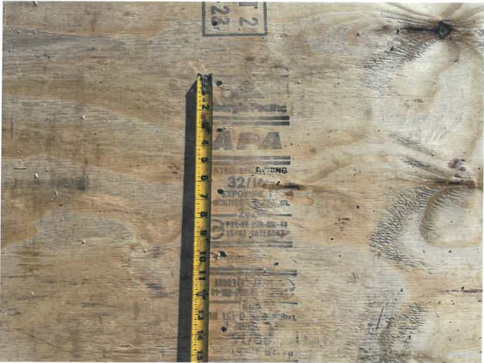
Figure 3 – Sheathing Fastener Field Spacing
