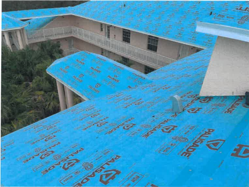
Figure 7 - Secondary Water Resistance
