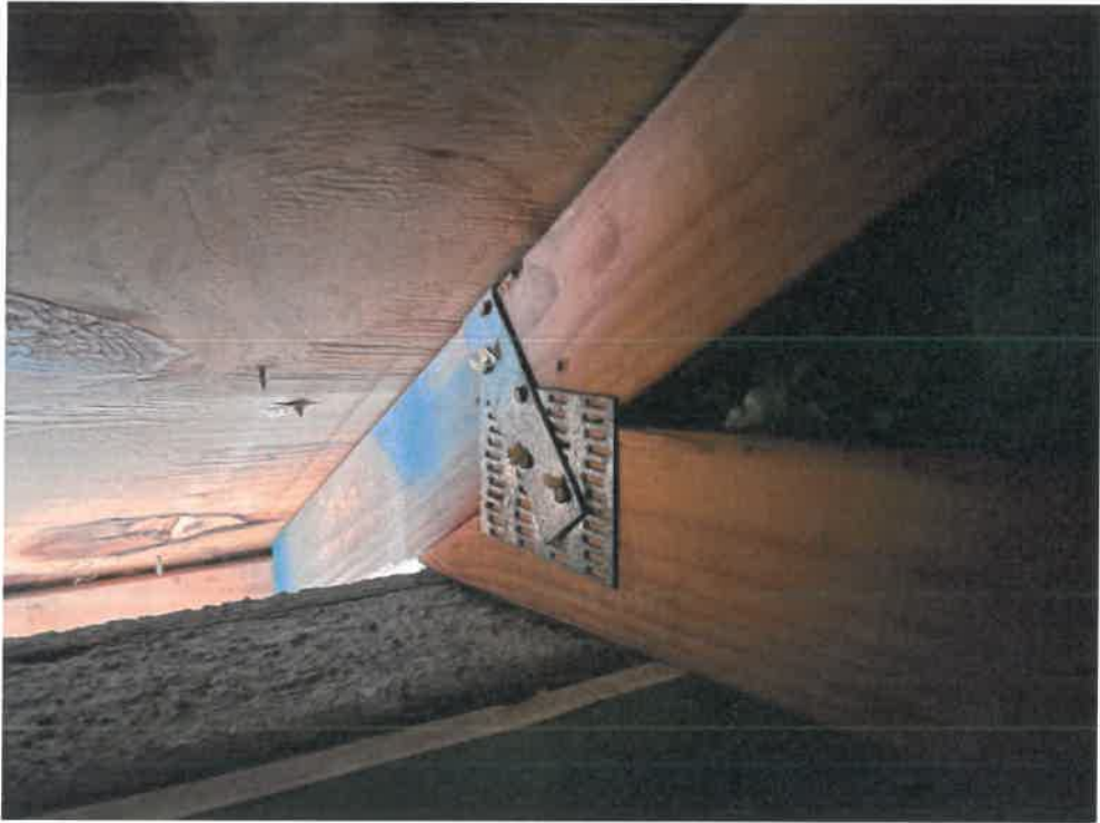
Figure 6 - Roof to Wall Attachment (Side 2)
