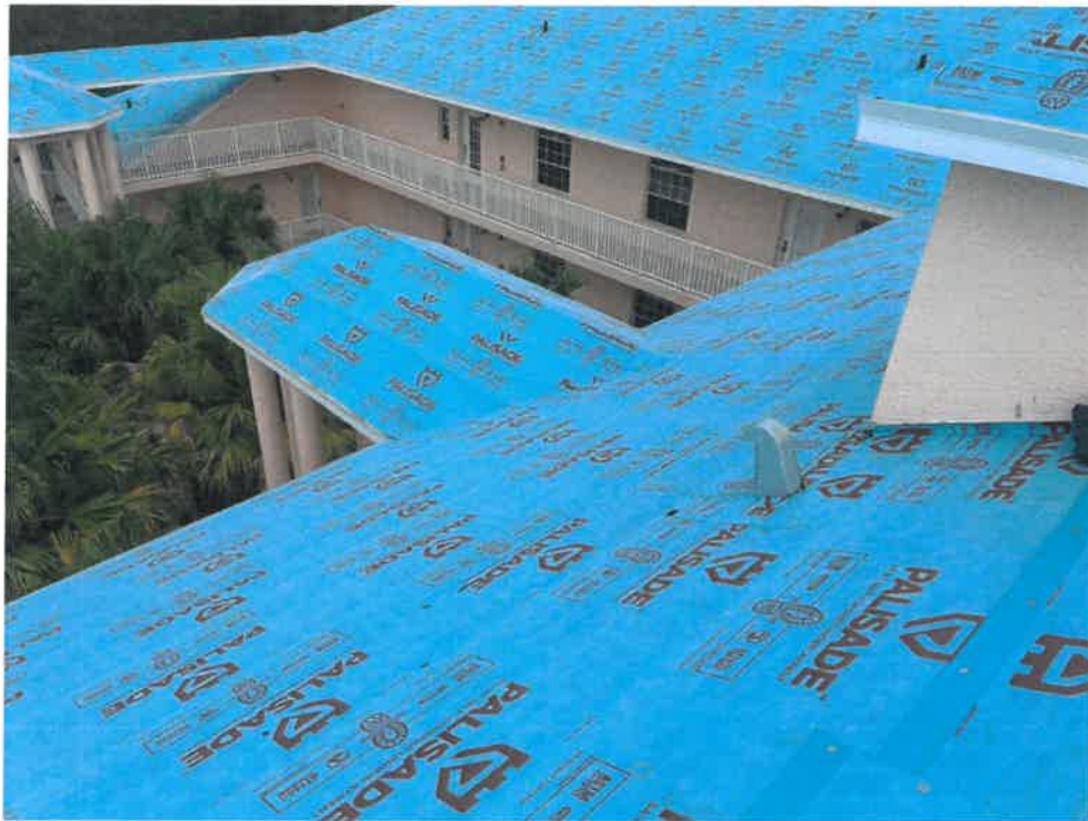
Figure 7 - Secondary Water Resistance
