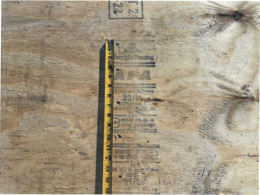
Figure 3 – Sheathing Fastener Field Spacing
