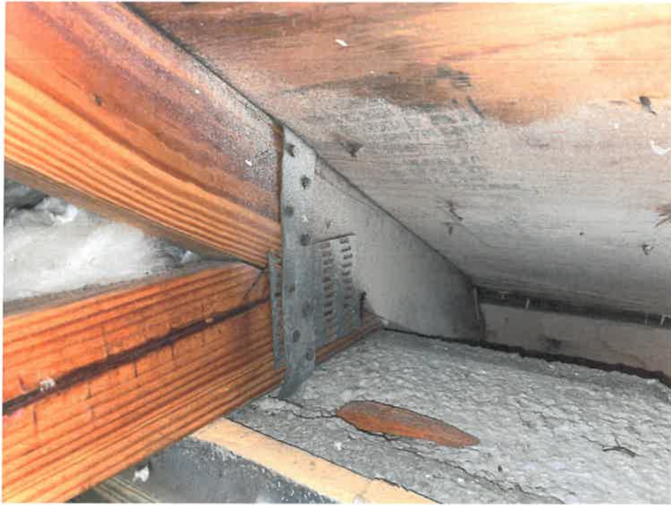
Figure 5 – Roof to Wall Attachment (Side 1)
