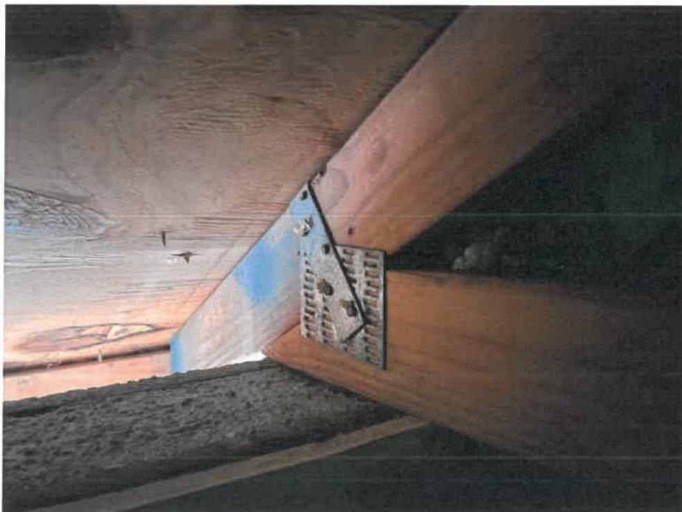
Figure 6 - Roof to Wall Attachment (Side 2)
