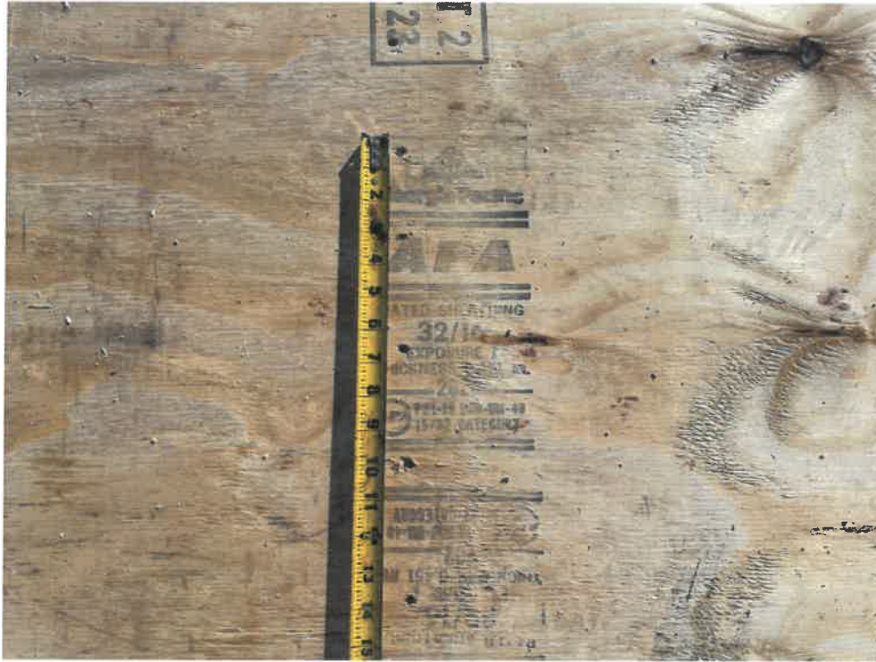
Figure 3 – Sheathing Fastener Field Spacing
