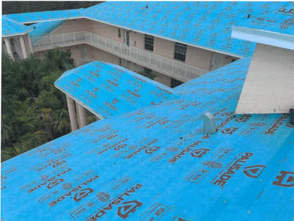
Figure 7 - Secondary Water Resistance
