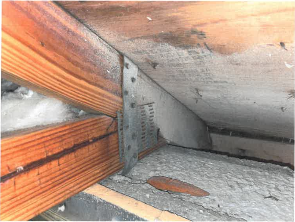
Figure 5 – Roof to Wall Attachment (Side 1)
