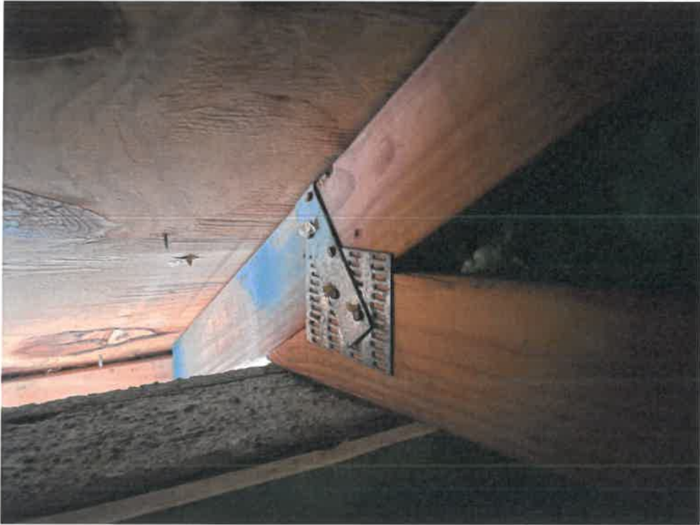
Figure 6 - Roof to Wall Attachment (Side 2)
