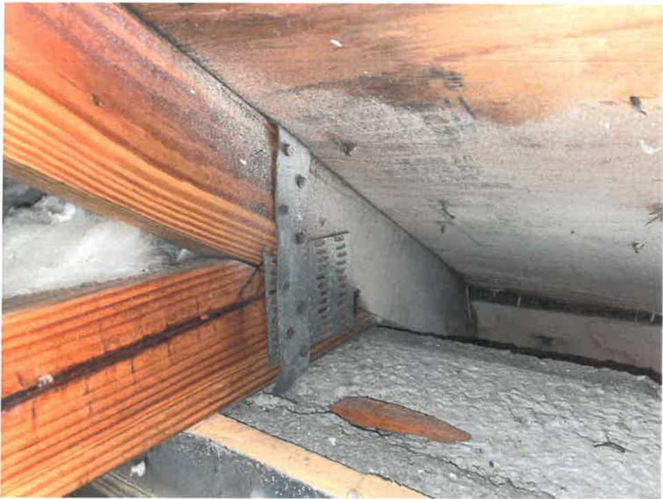
Figure 5 – Roof to Wall Attachment (Side 1)
