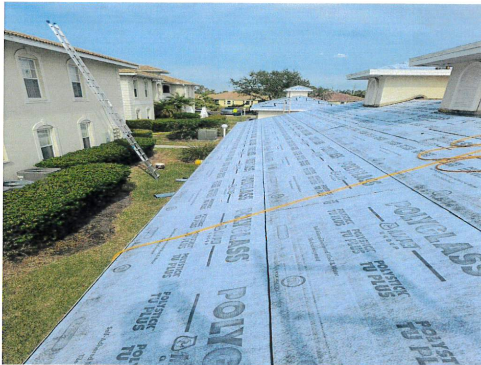
Figure 7 – Secondary Water Resistance
