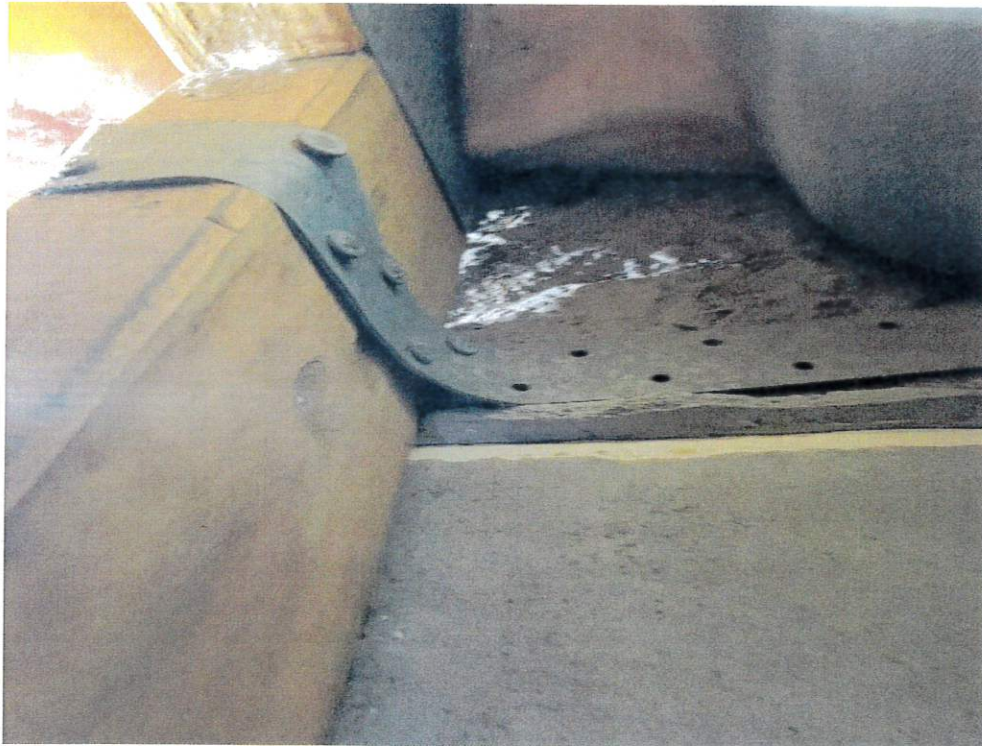
Figure 6 - Roof to Wall Attachment
