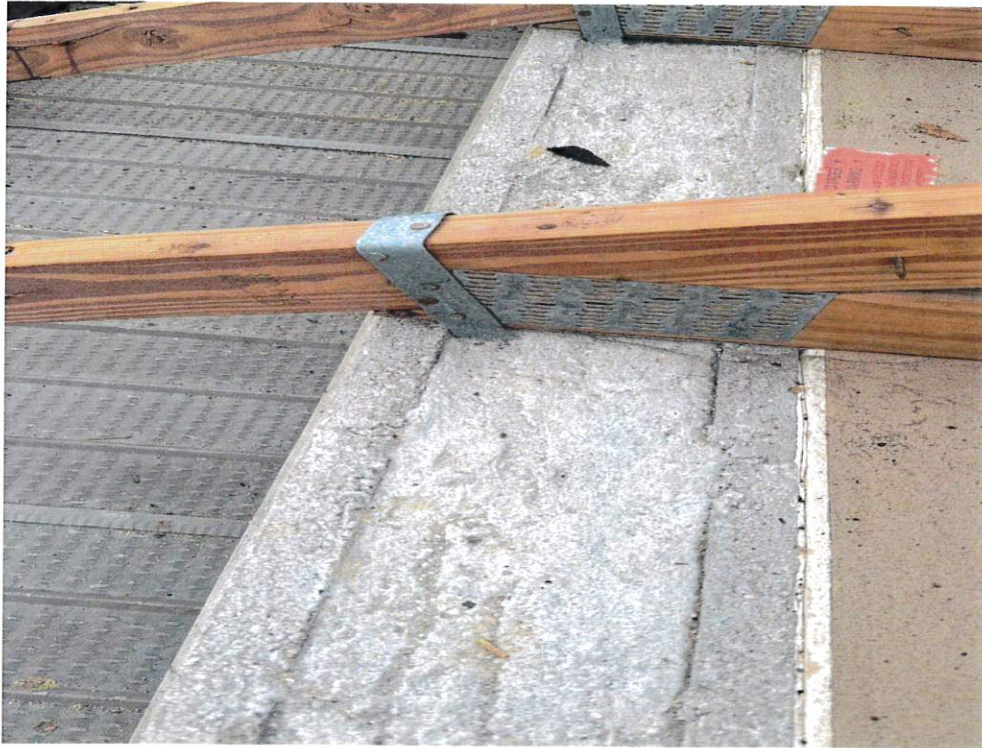
Figure 5 – Roof to Wall Attachment
