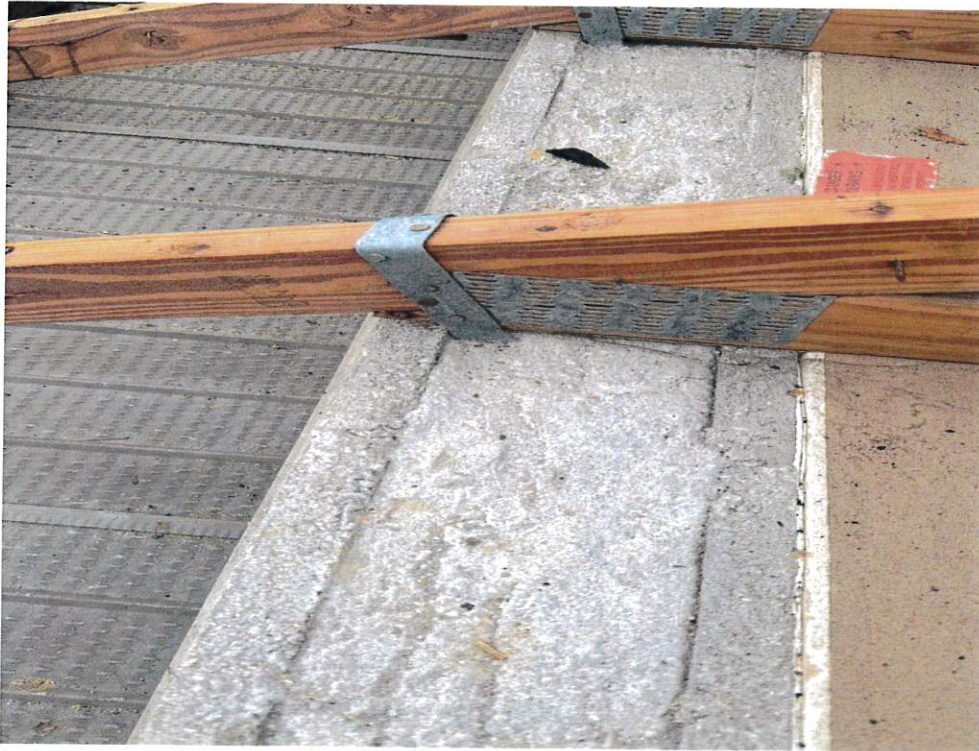
Figure 5 – Roof to Wall Attachment
