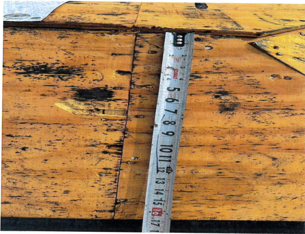
Figure 3 – Sheathing Fastener Spacing
