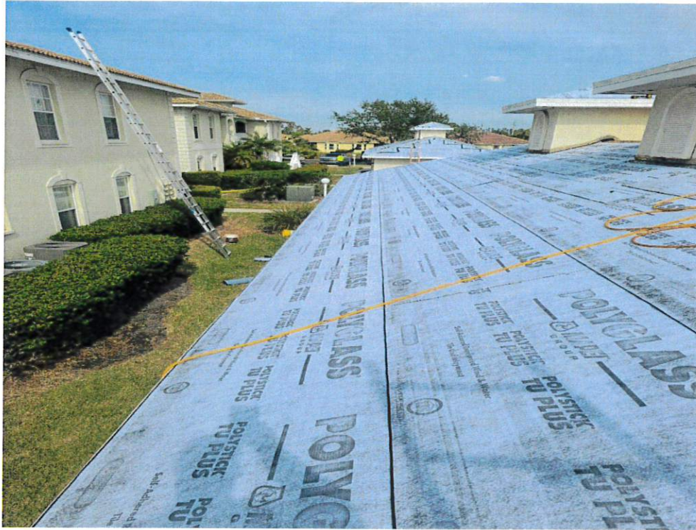
Figure 7 – Secondary Water Resistance
