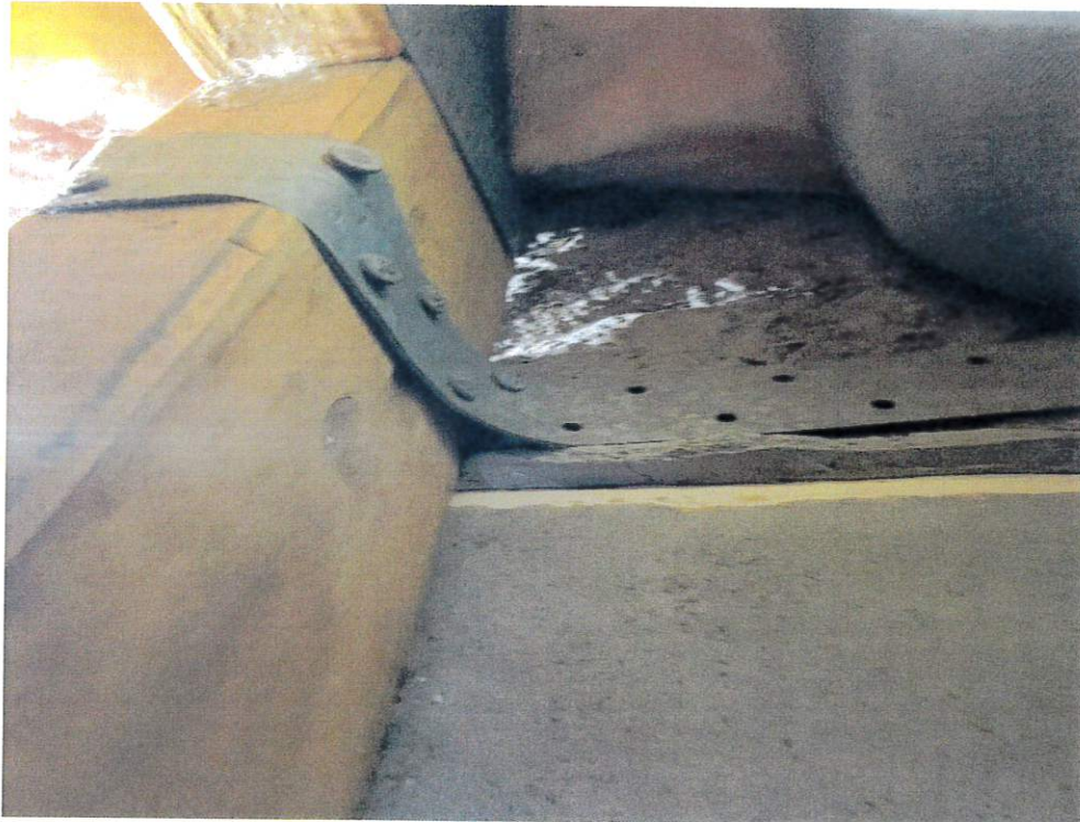
Figure 6 - Roof to Wall Attachment
