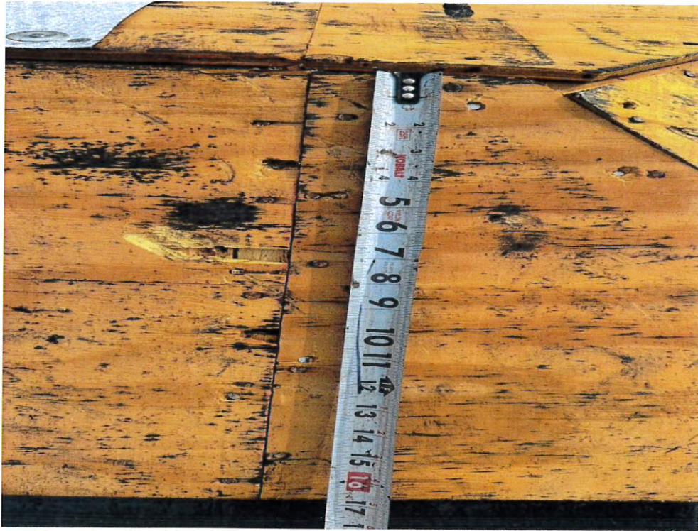
Figure 3 – Sheathing Fastener Spacing
