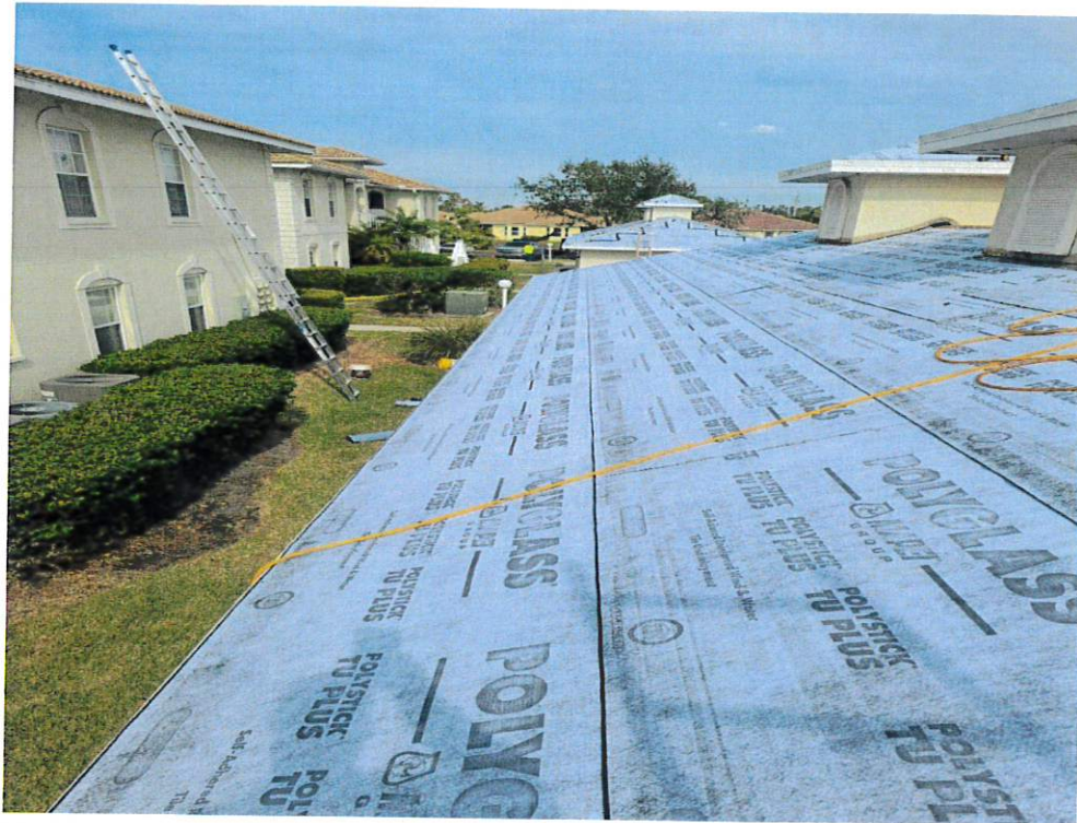
Figure 7 – Secondary Water Resistance
