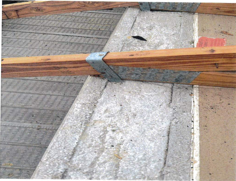
Figure 5 – Roof to Wall Attachment
