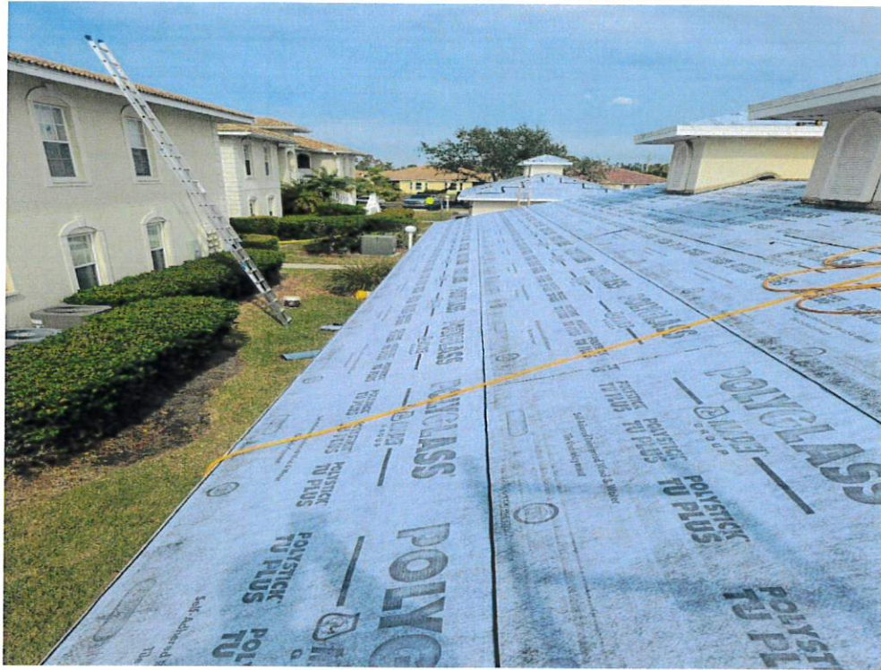
Figure 7 – Secondary Water Resistance
