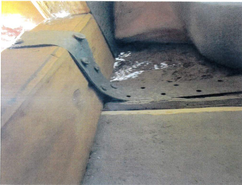
Figure 6 - Roof to Wall Attachment
