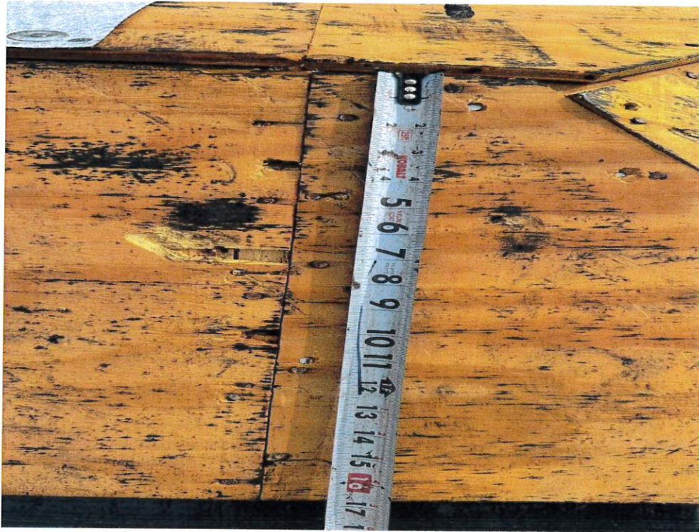
Figure 3 – Sheathing Fastener Spacing
