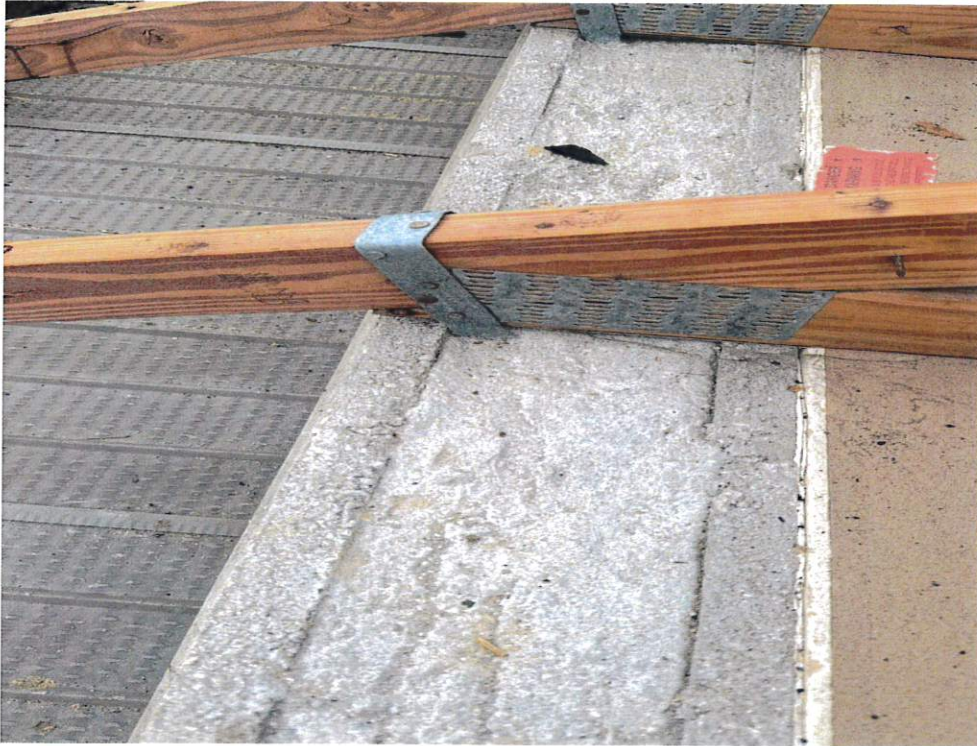
Figure 5 – Roof to Wall Attachment
