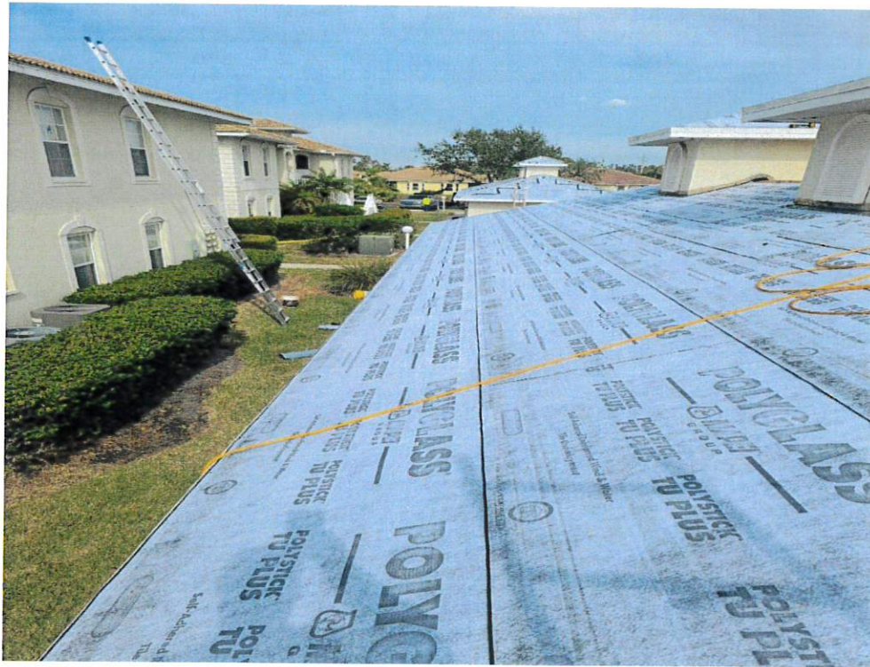
Figure 7 – Secondary Water Resistance
