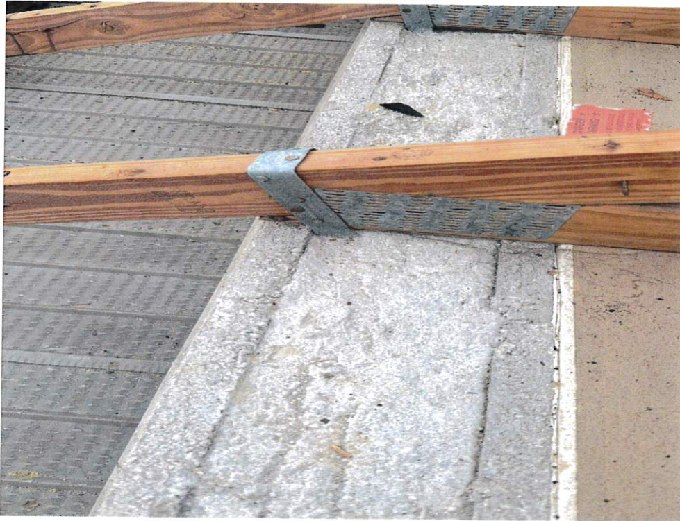
Figure 5 – Roof to Wall Attachment
