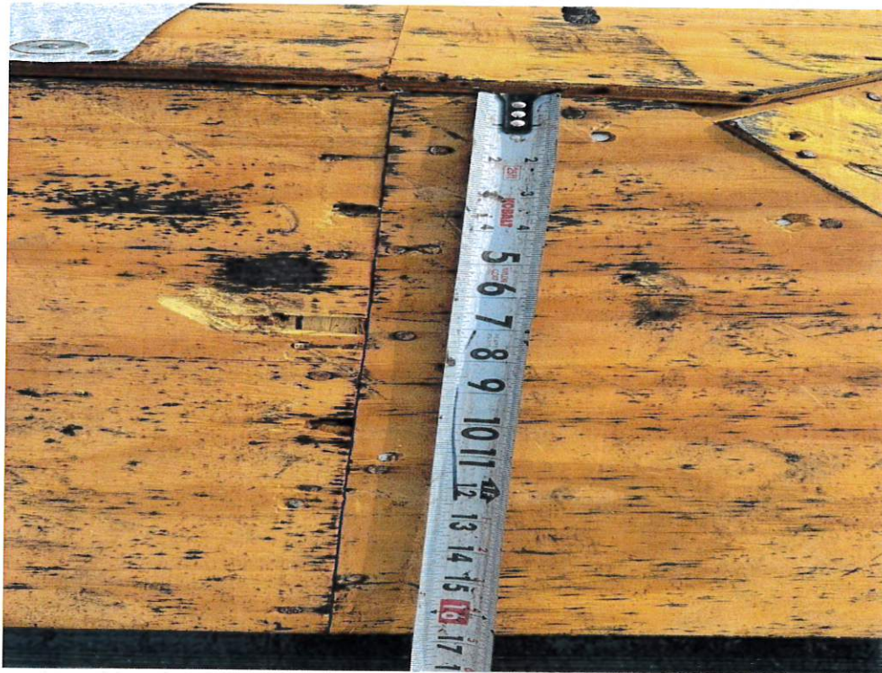
Figure 3 – Sheathing Fastener Spacing
