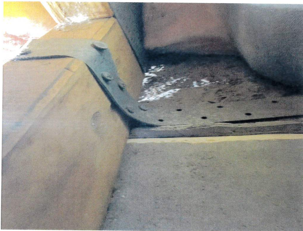
Figure 6 - Roof to Wall Attachment
