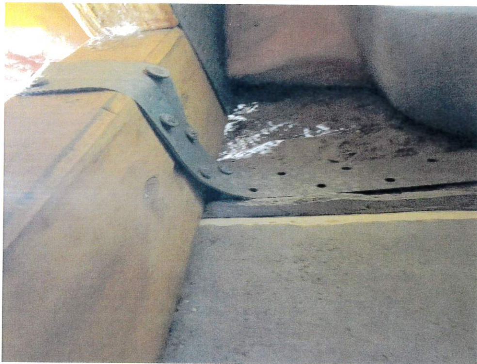
Figure 6 - Roof to Wall Attachment
