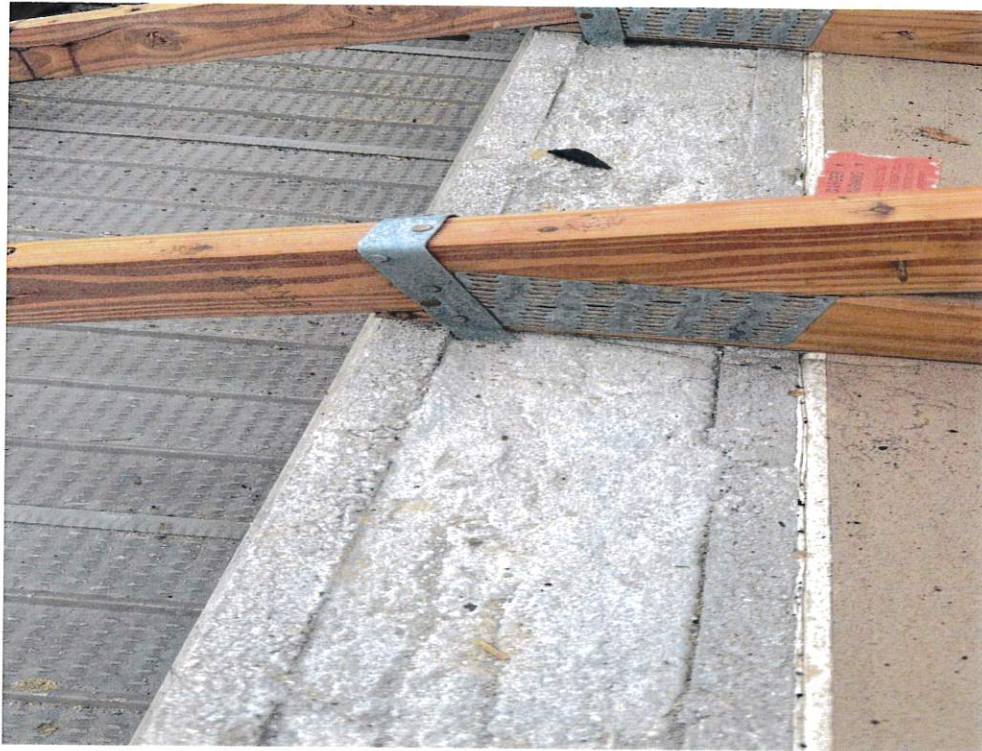
Figure 5 – Roof to Wall Attachment
