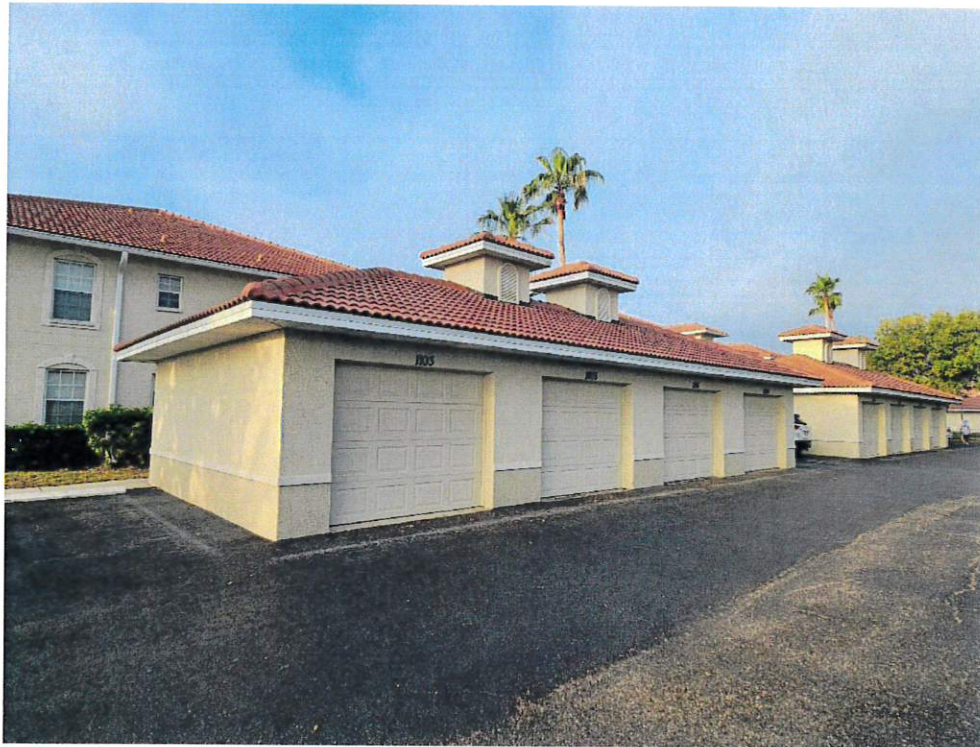
Figure 1: Roof Type (Concrete Barrel Tile) and Geometry (Hip)
