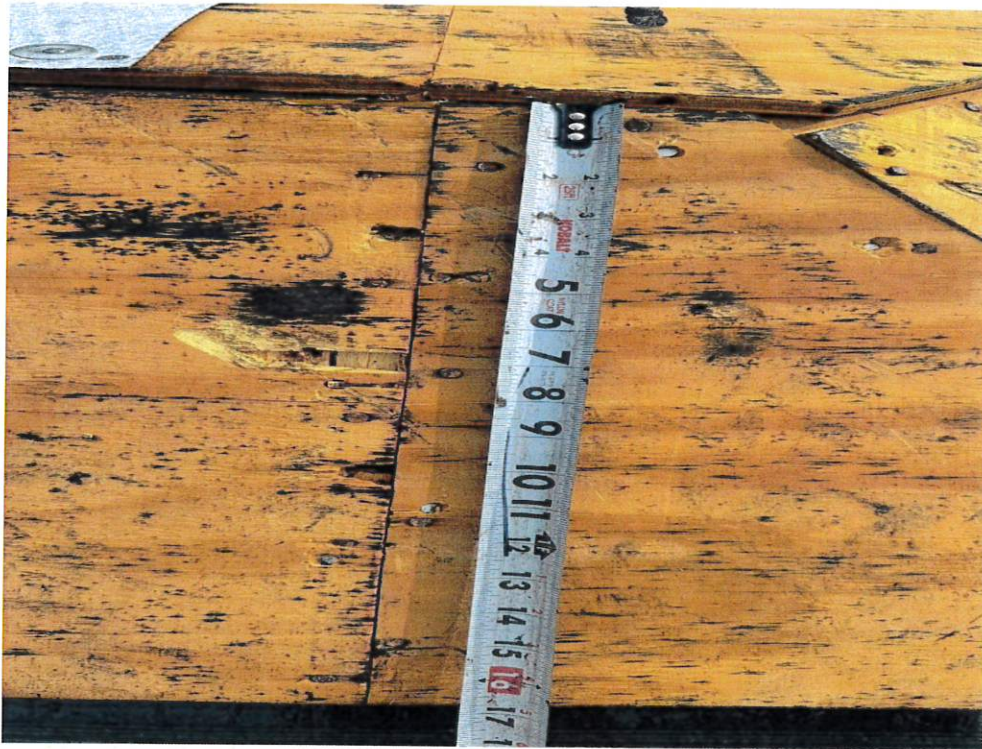
Figure 3 – Sheathing Fastener Spacing
