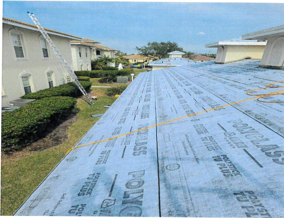
Figure 7 – Secondary Water Resistance
