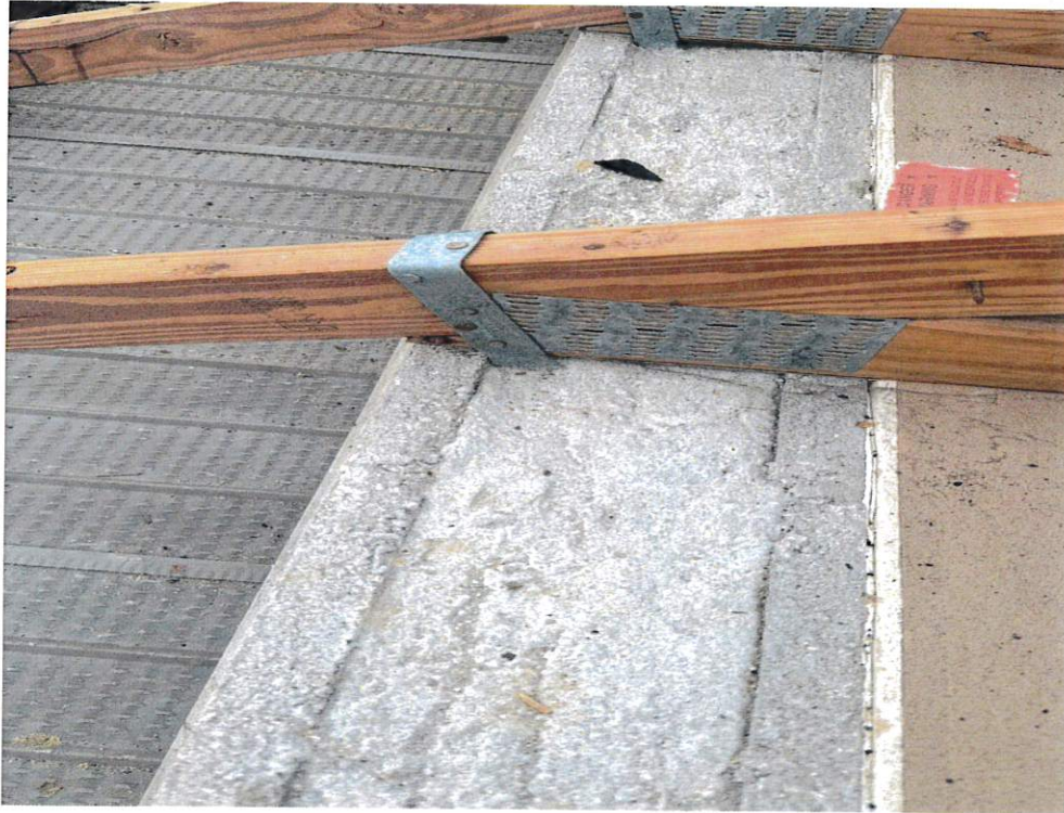
Figure 5 – Roof to Wall Attachment
