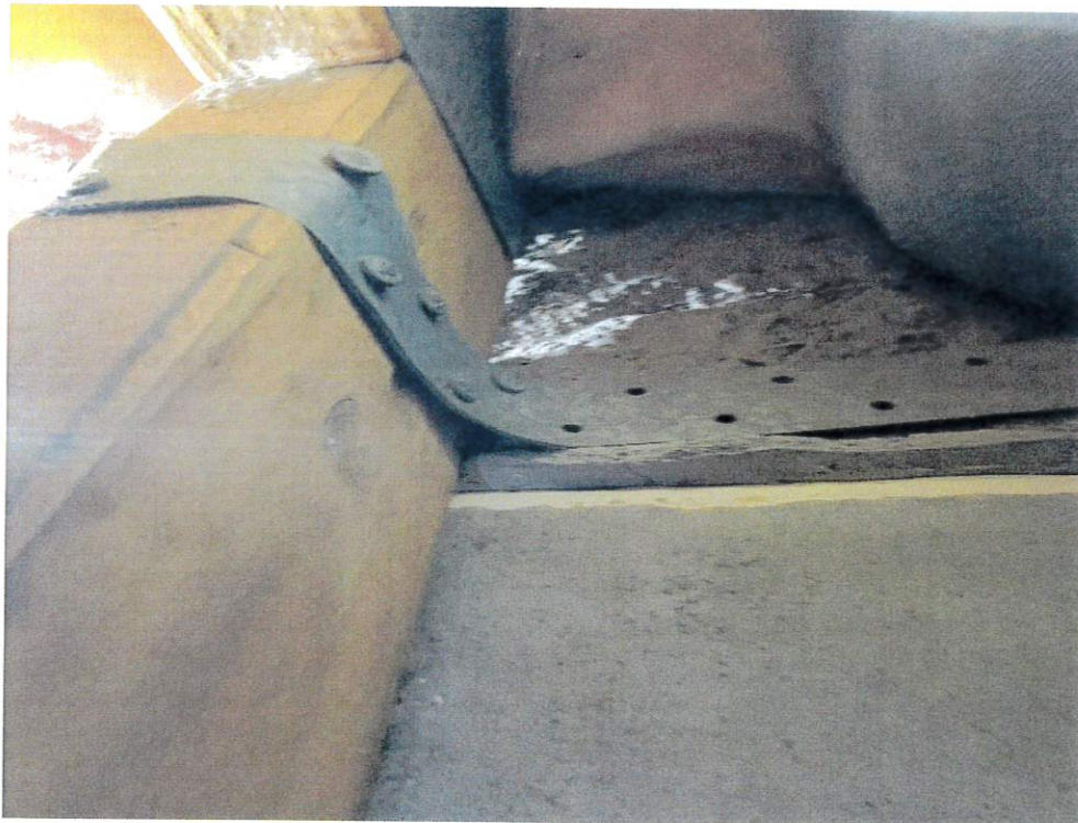
Figure 6 - Roof to Wall Attachment
