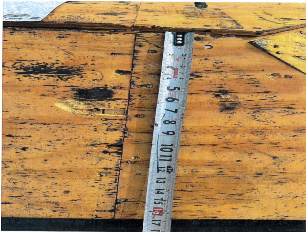
Figure 3 – Sheathing Fastener Spacing
