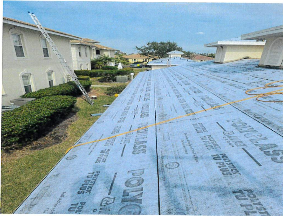
Figure 7 – Secondary Water Resistance
