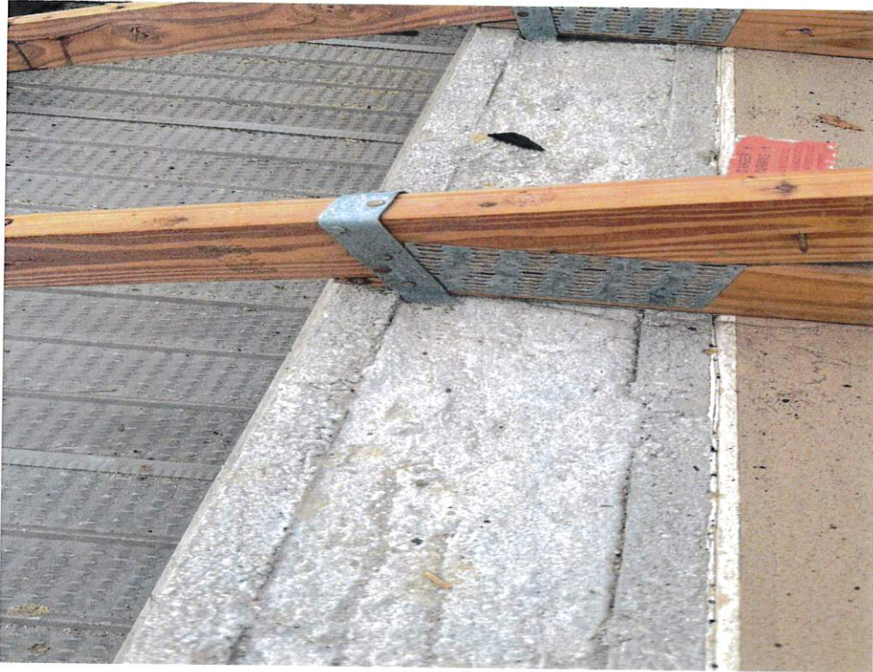
Figure 5 – Roof to Wall Attachment
