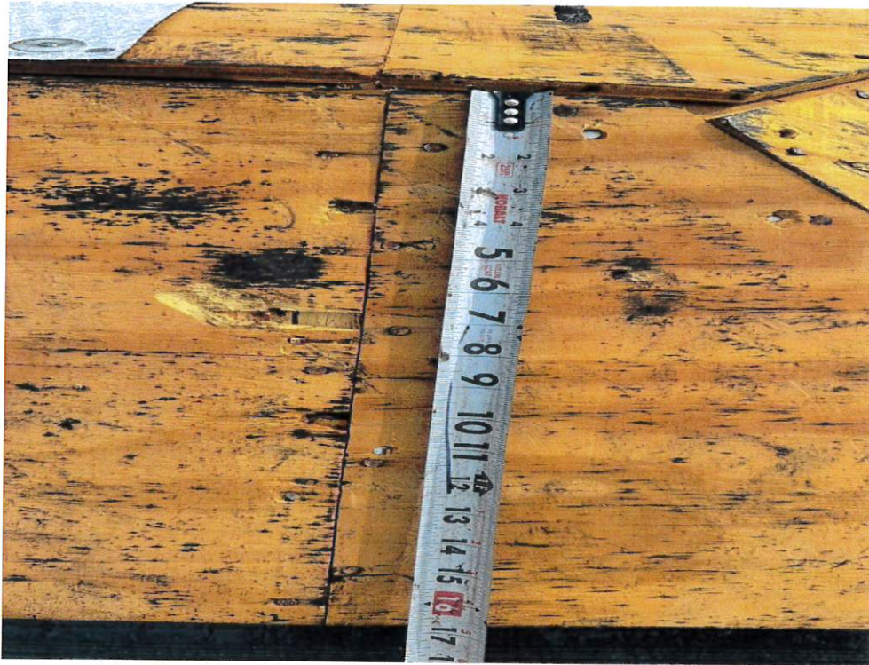
Figure 3 – Sheathing Fastener Spacing
