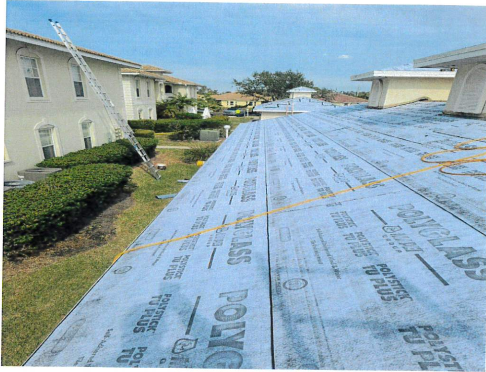
Figure 7 – Secondary Water Resistance
