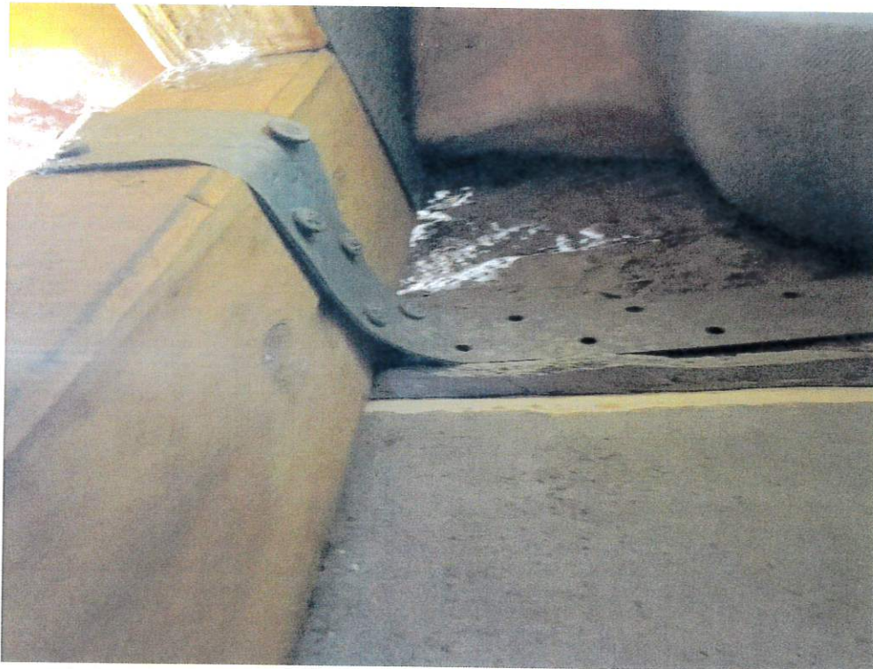
Figure 6 - Roof to Wall Attachment
