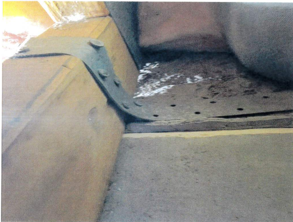
Figure 6 - Roof to Wall Attachment
