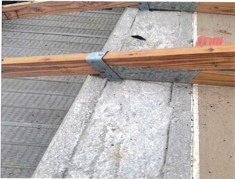
Figure 5 – Roof to Wall Attachment
