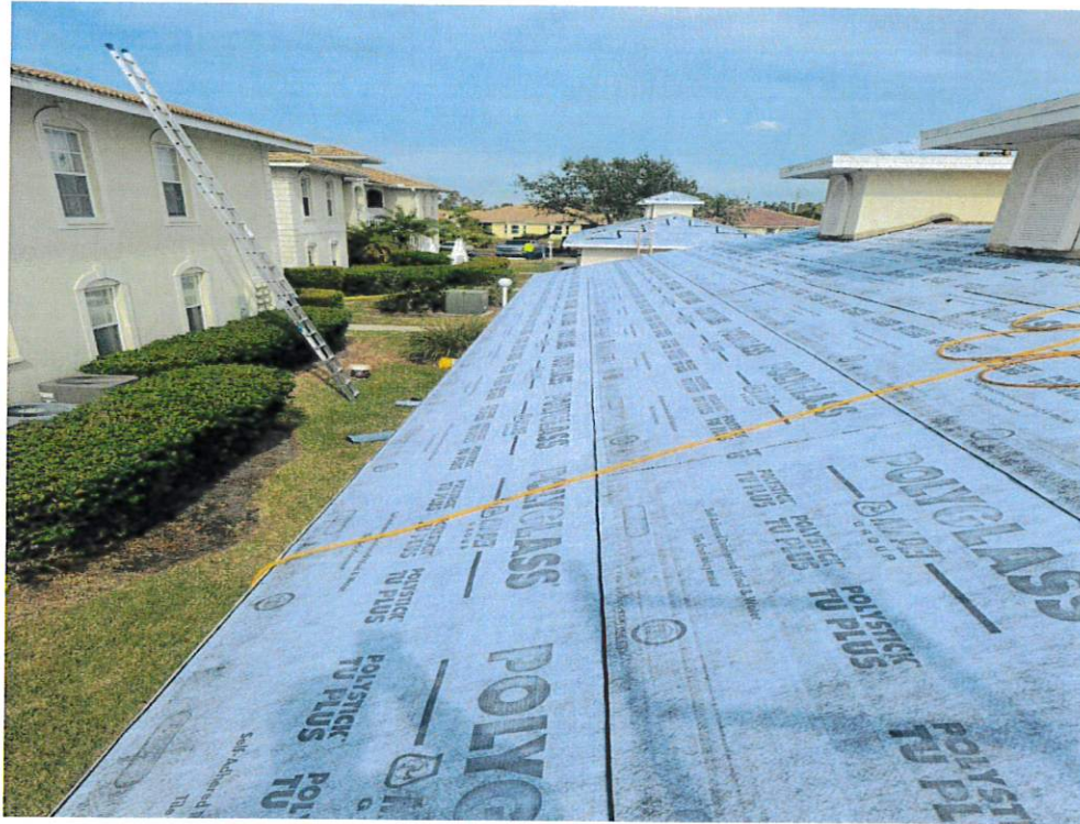
Figure 7 – Secondary Water Resistance
