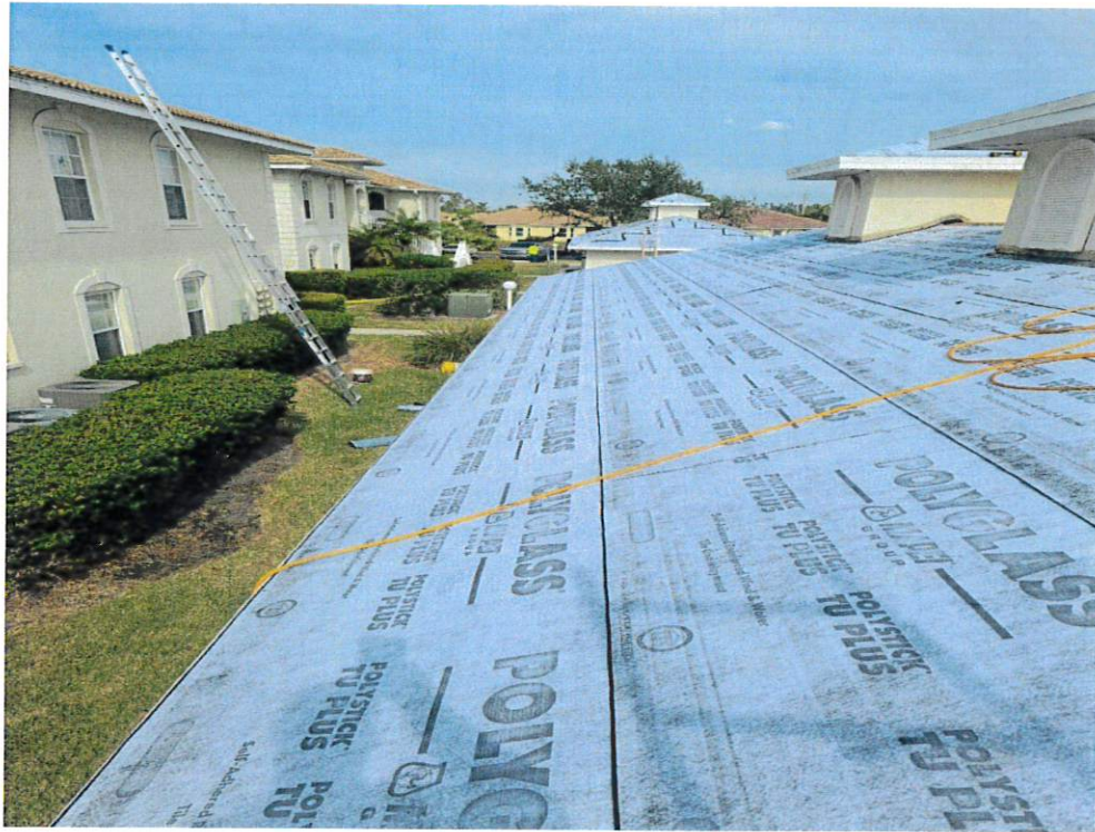
Figure 7 – Secondary Water Resistance
