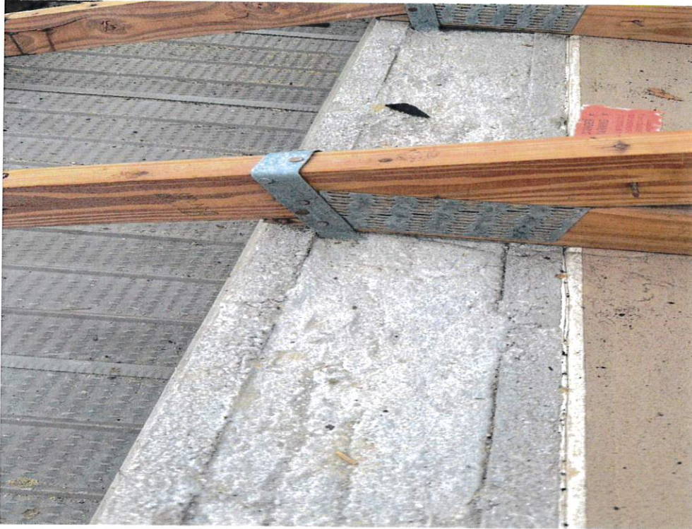
Figure 5 – Roof to Wall Attachment
