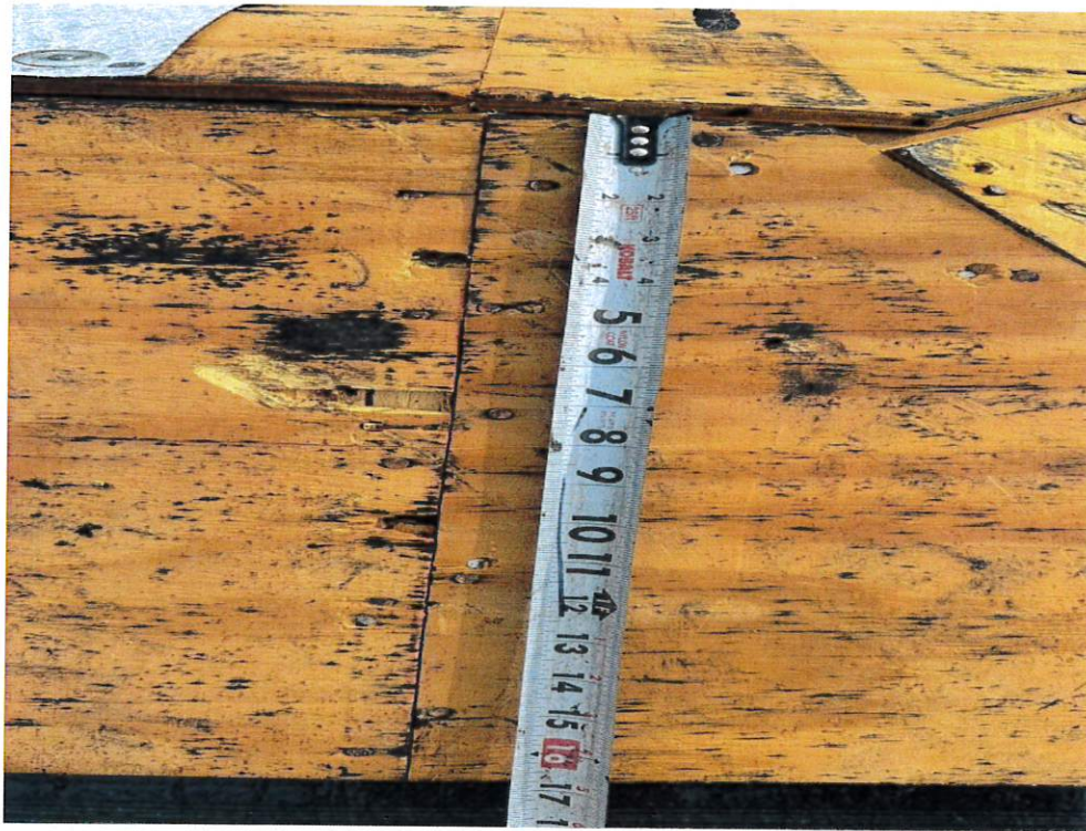
Figure 3 – Sheathing Fastener Spacing
