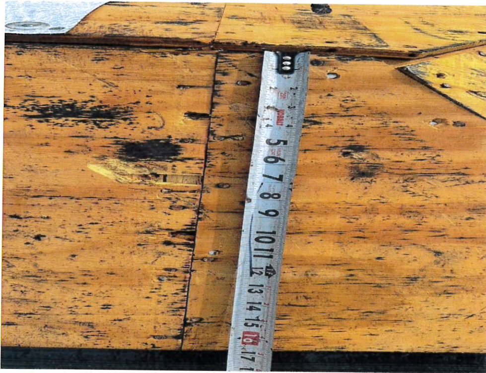
Figure 3 – Sheathing Fastener Spacing
