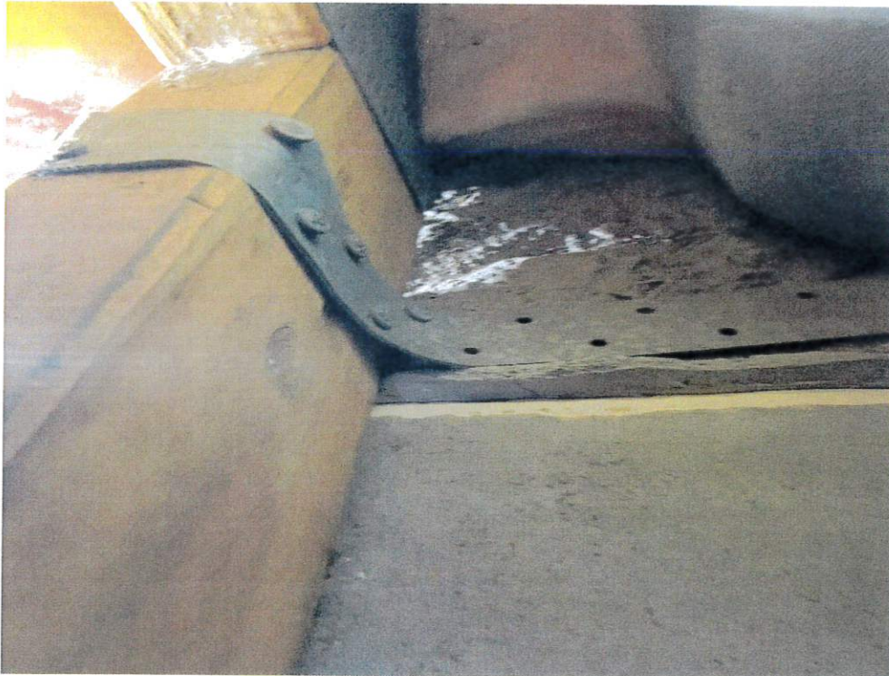
Figure 6 - Roof to Wall Attachment
