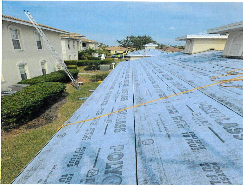
Figure 7 – Secondary Water Resistance
