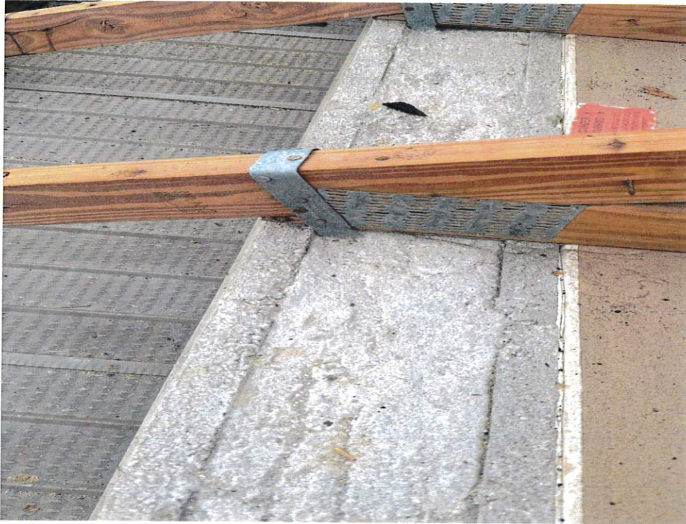
Figure 5 – Roof to Wall Attachment
