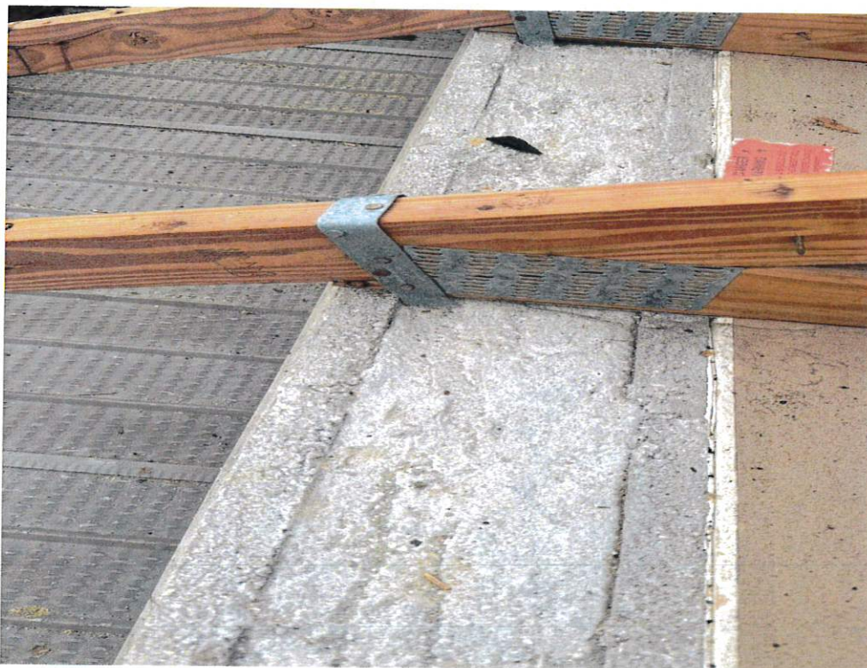
Figure 5 – Roof to Wall Attachment
