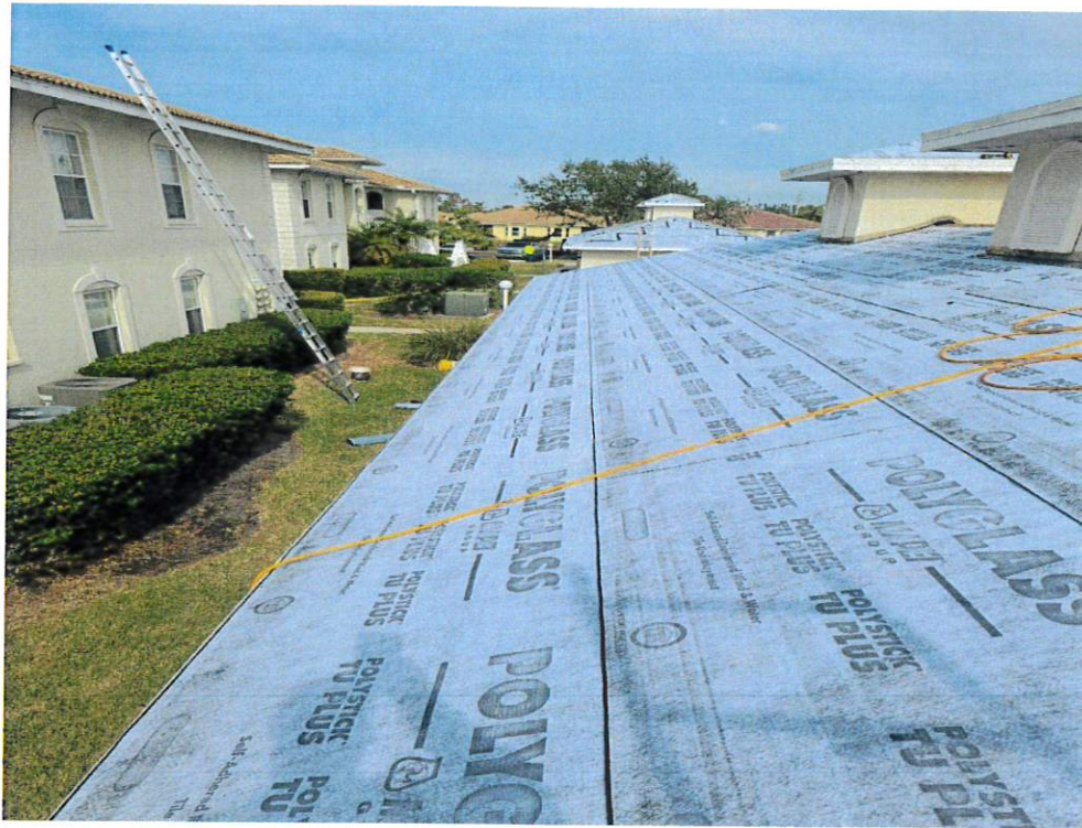
Figure 7 – Secondary Water Resistance
