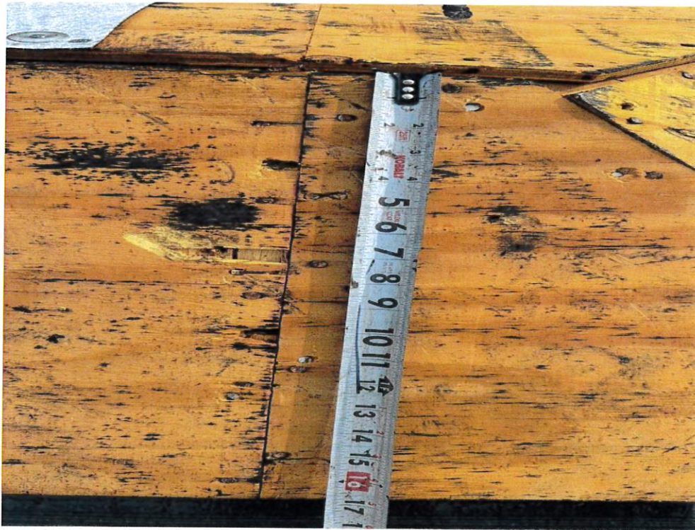
Figure 3 – Sheathing Fastener Spacing
