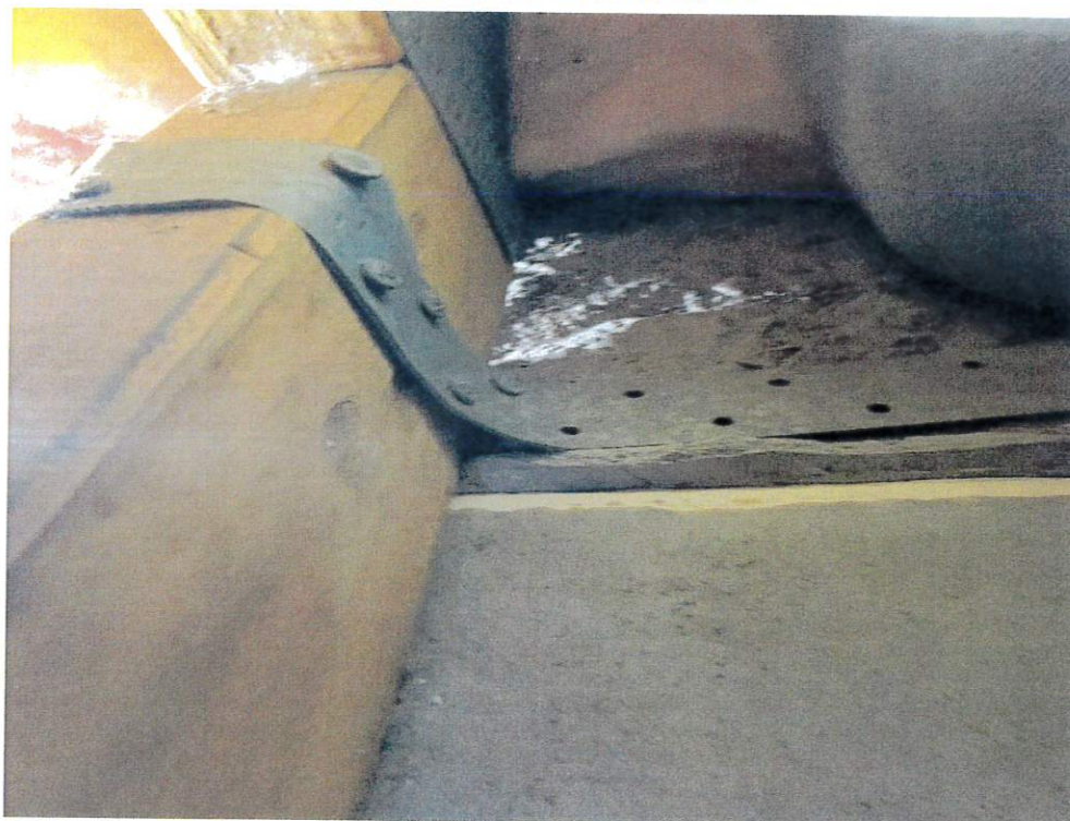
Figure 6 - Roof to Wall Attachment
