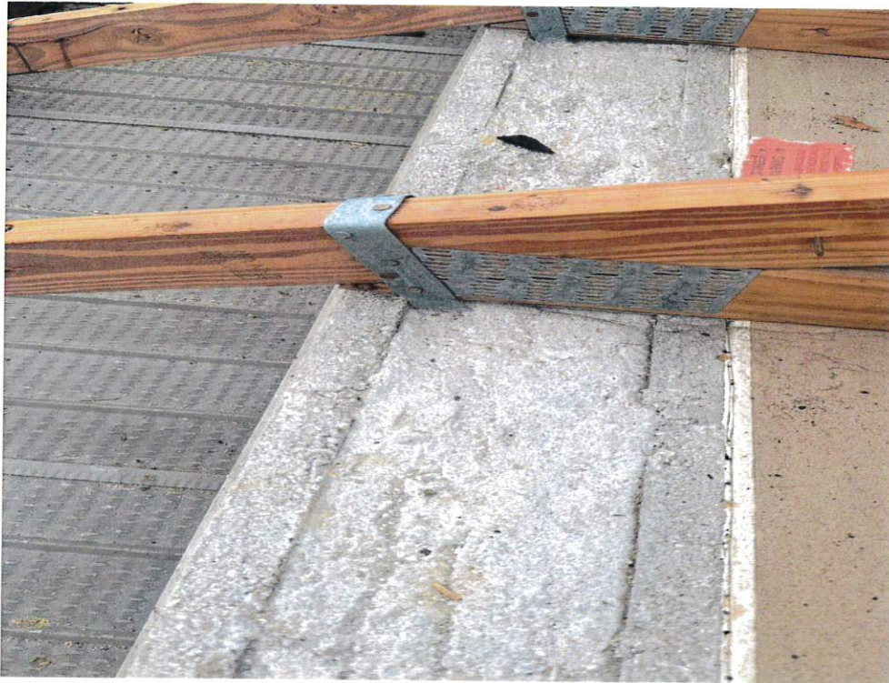
Figure 5 – Roof to Wall Attachment
