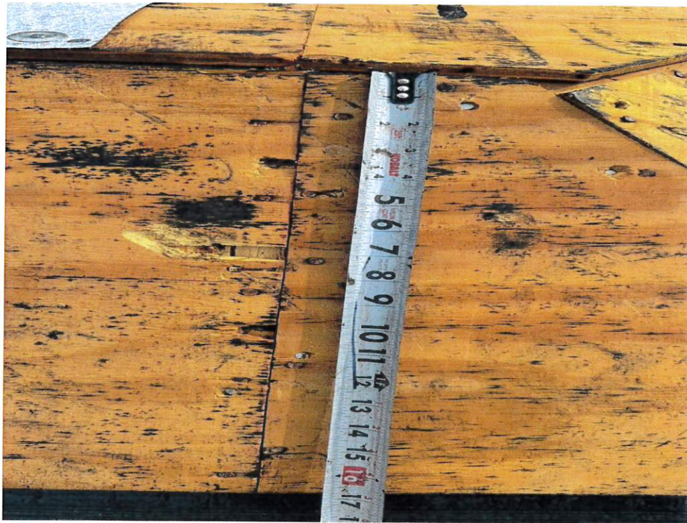
Figure 3 – Sheathing Fastener Spacing
