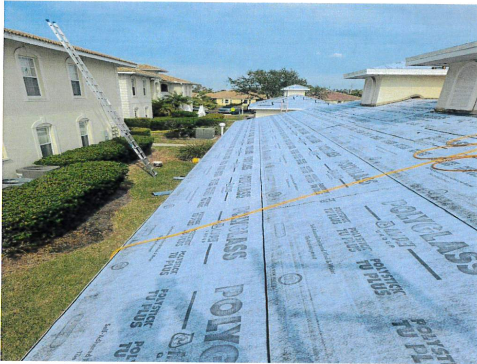
Figure 7 – Secondary Water Resistance
