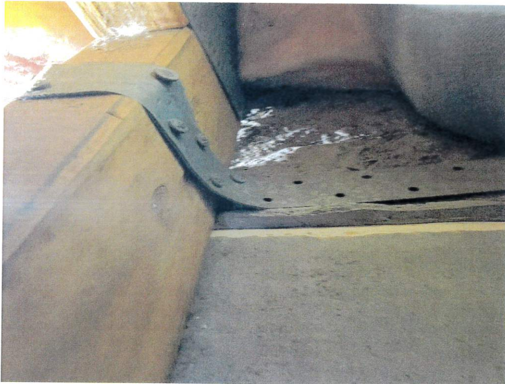
Figure 6 - Roof to Wall Attachment
