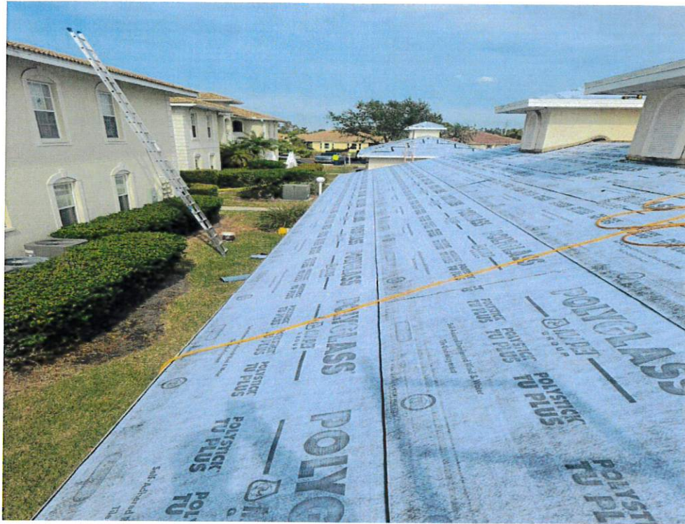
Figure 7 – Secondary Water Resistance
