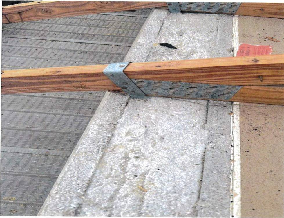
Figure 5 – Roof to Wall Attachment
