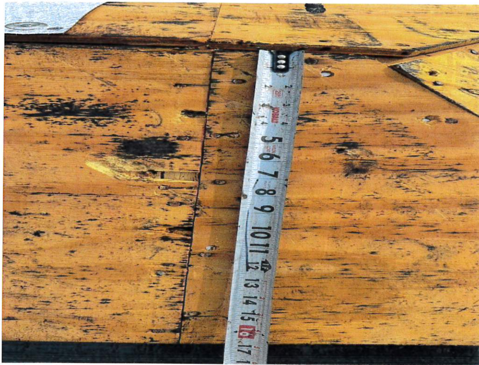
Figure 3 – Sheathing Fastener Spacing
