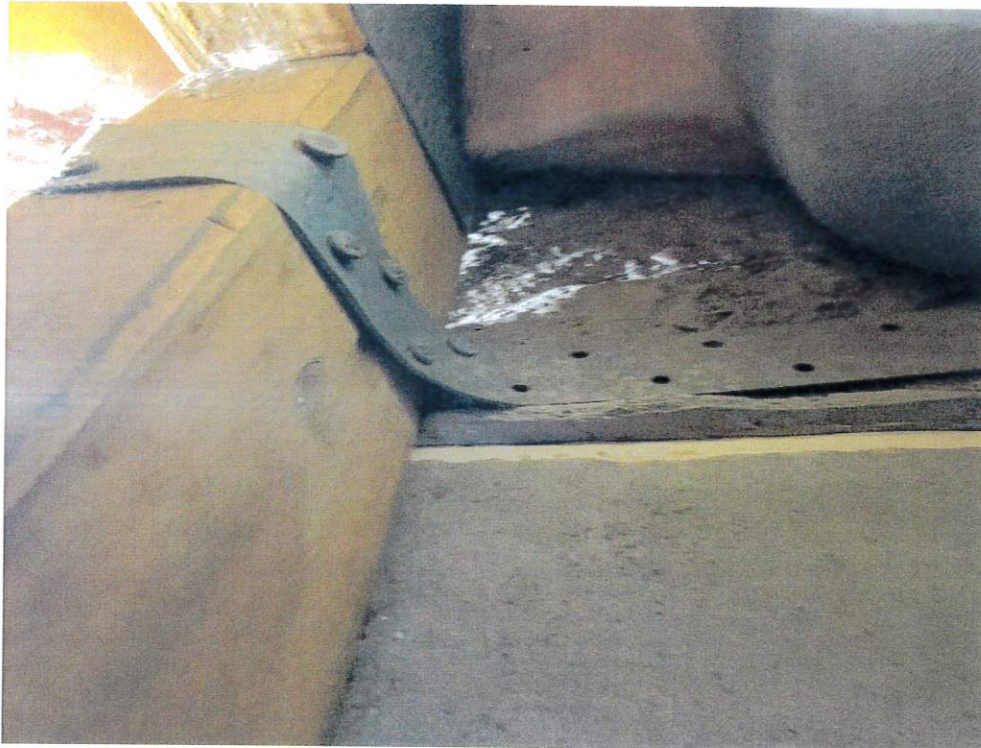
Figure 6 - Roof to Wall Attachment
