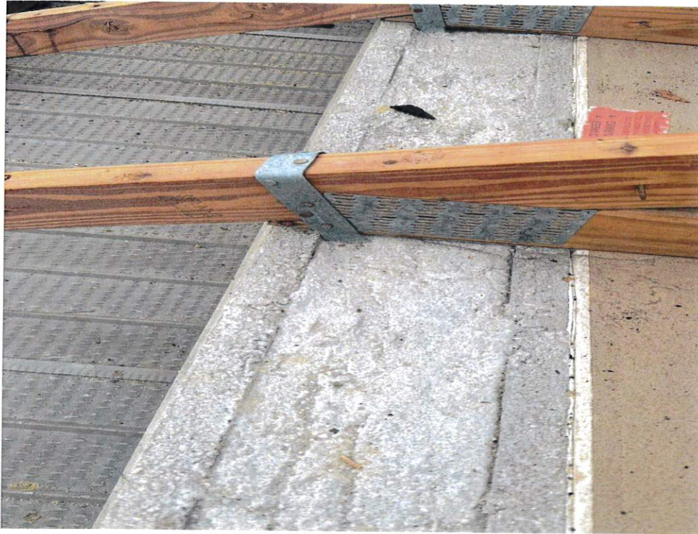
Figure 5 – Roof to Wall Attachment
