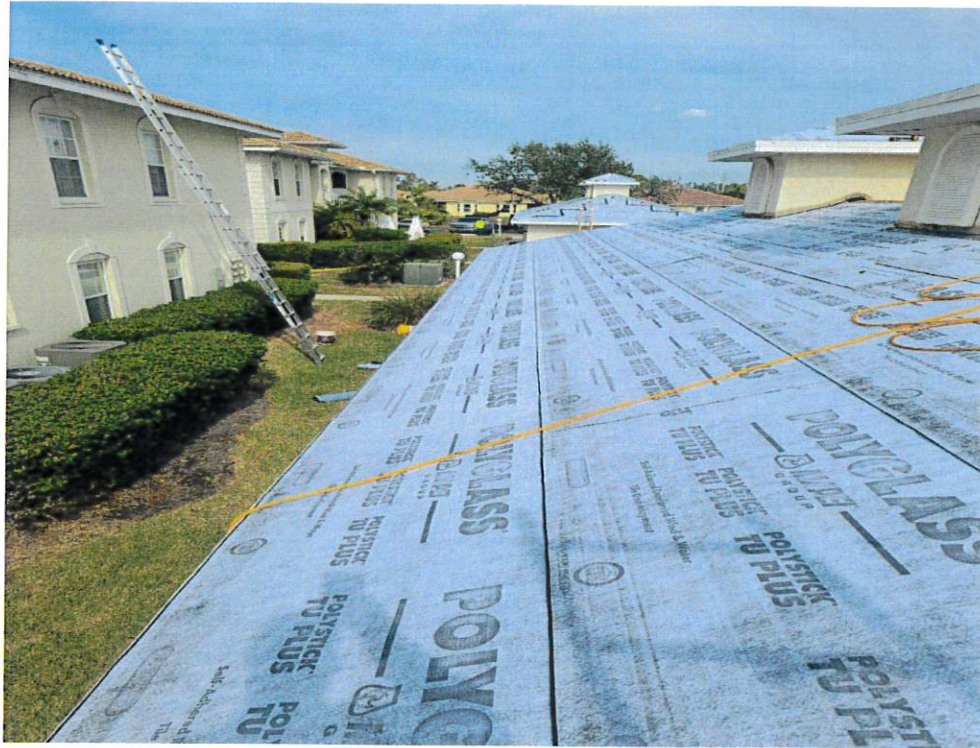
Figure 7 – Secondary Water Resistance
