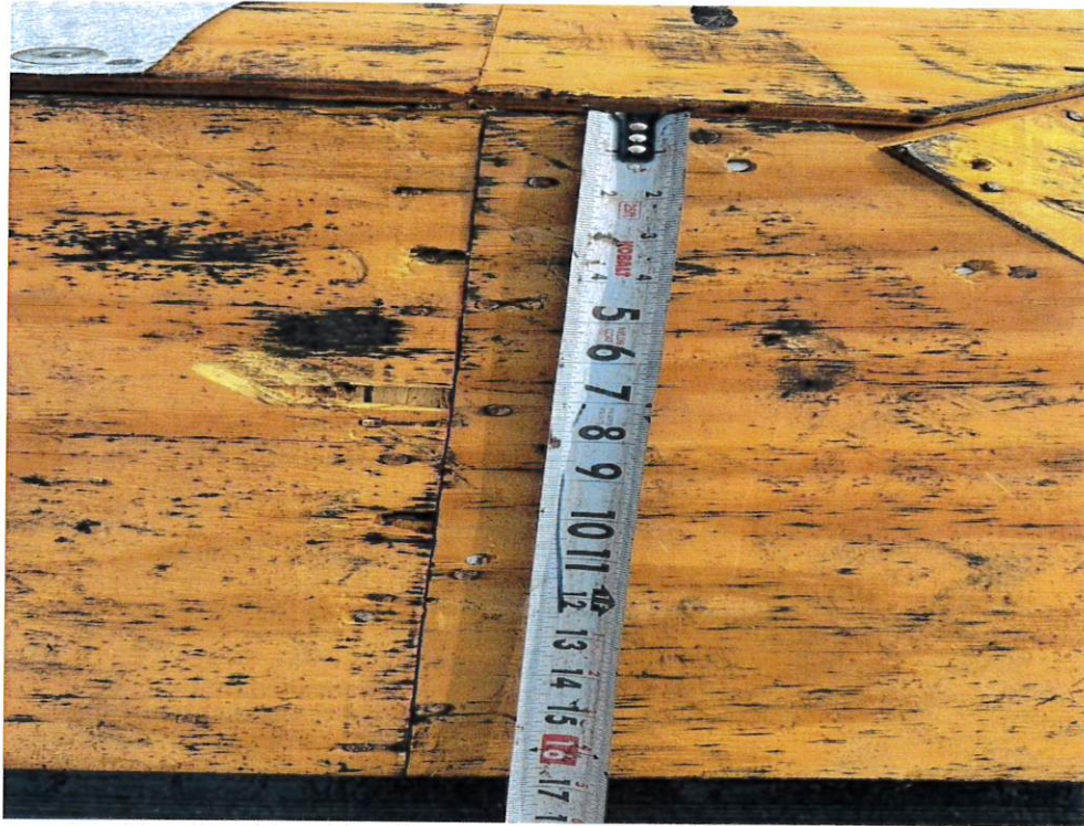
Figure 3 – Sheathing Fastener Spacing
