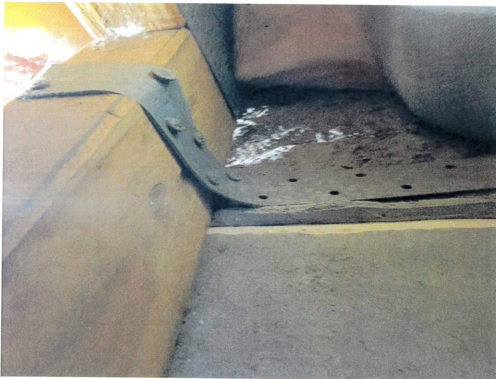
Figure 6 - Roof to Wall Attachment
