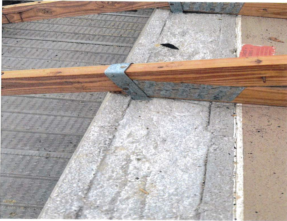
Figure 5 – Roof to Wall Attachment
