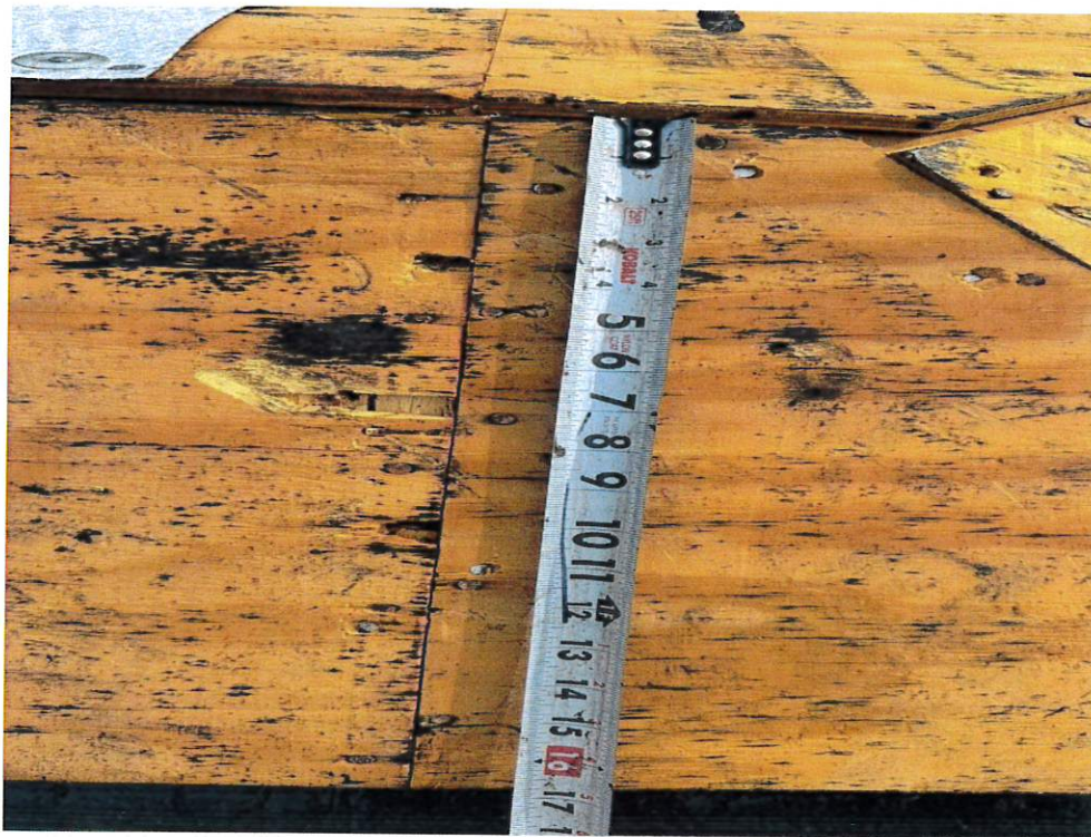
Figure 3 – Sheathing Fastener Spacing
