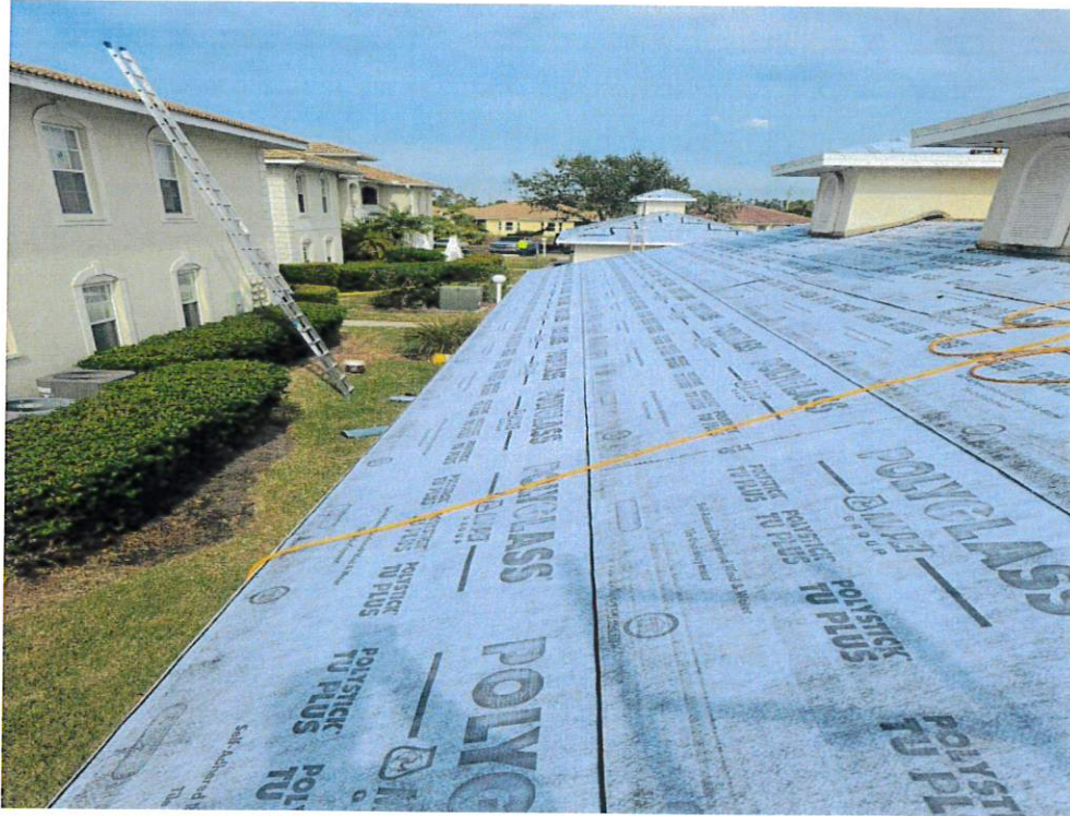
Figure 7 – Secondary Water Resistance
