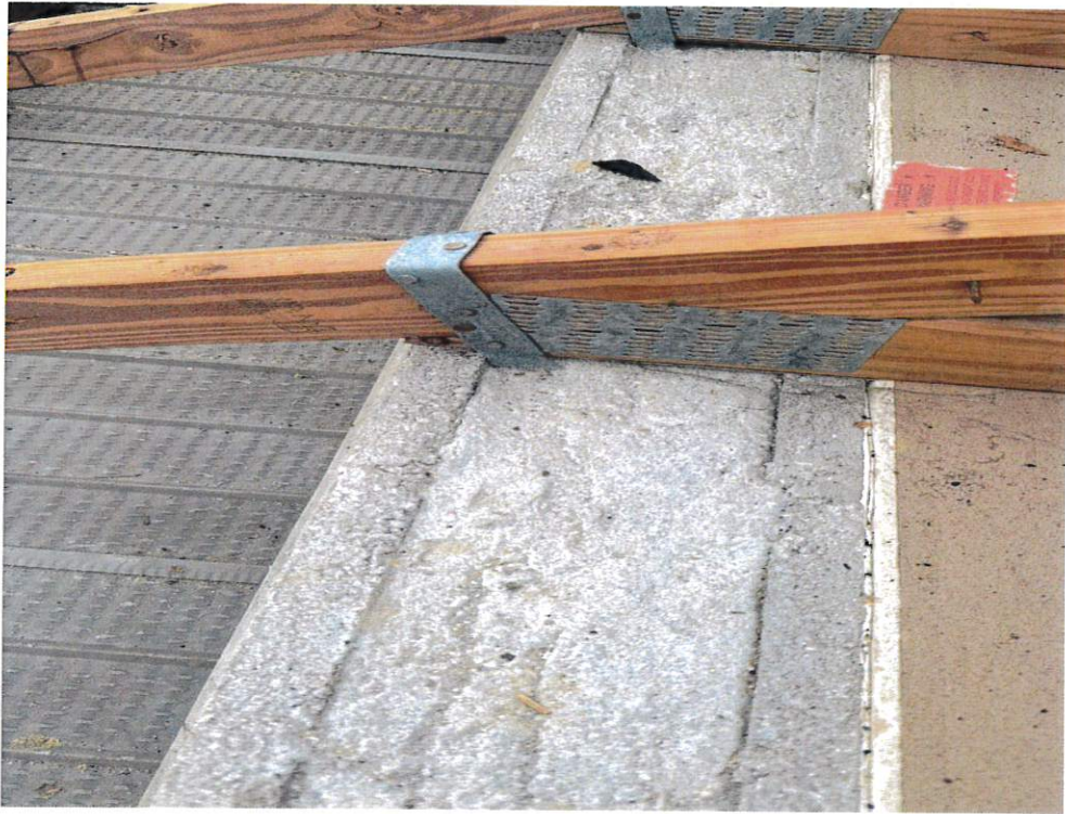
Figure 5 – Roof to Wall Attachment
