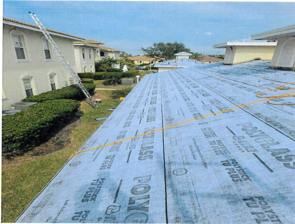
Figure 7 – Secondary Water Resistance
