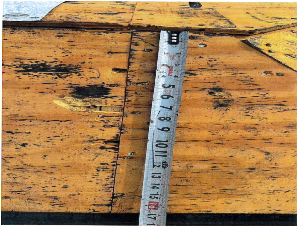
Figure 3 – Sheathing Fastener Spacing
