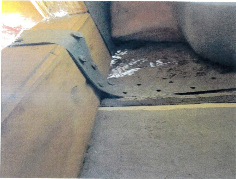
Figure 6 - Roof to Wall Attachment
