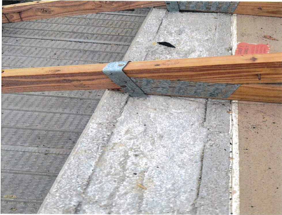
Figure 5 – Roof to Wall Attachment
