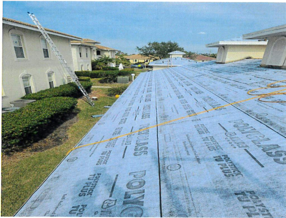
Figure 7 – Secondary Water Resistance
