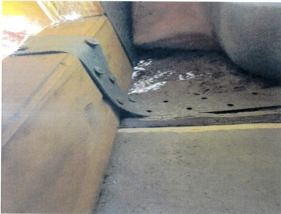
Figure 6 - Roof to Wall Attachment
