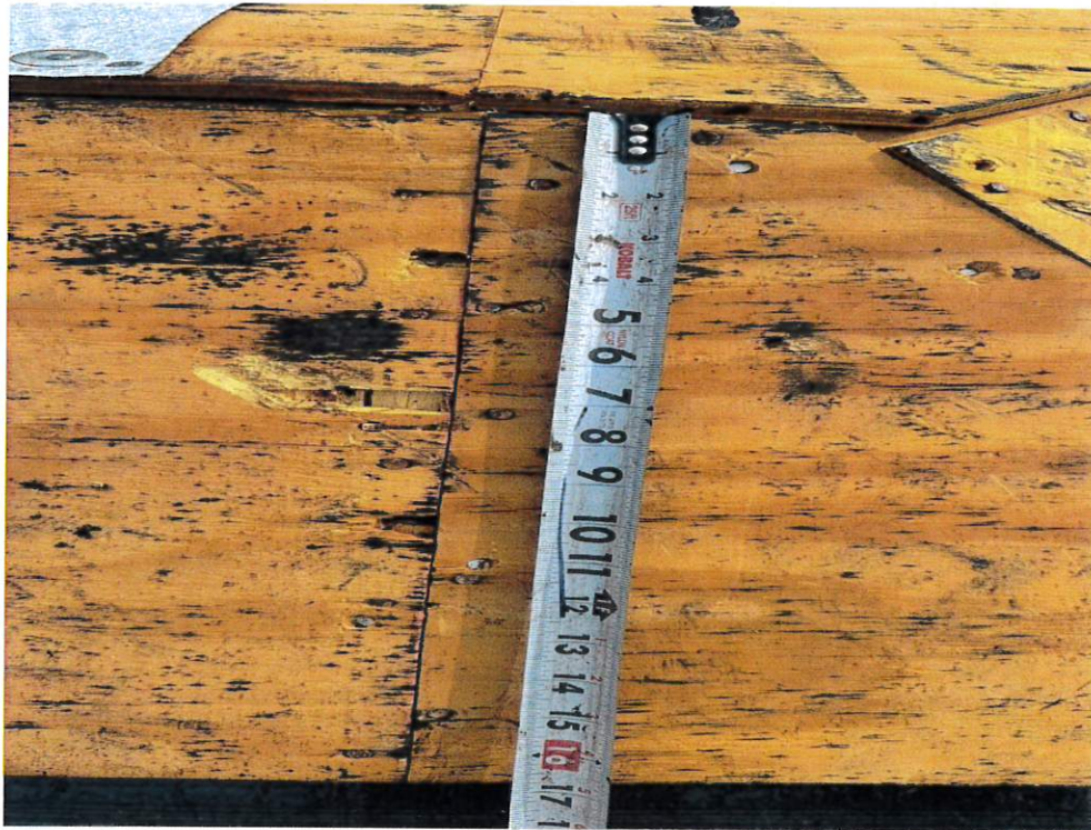
Figure 3 – Sheathing Fastener Spacing
