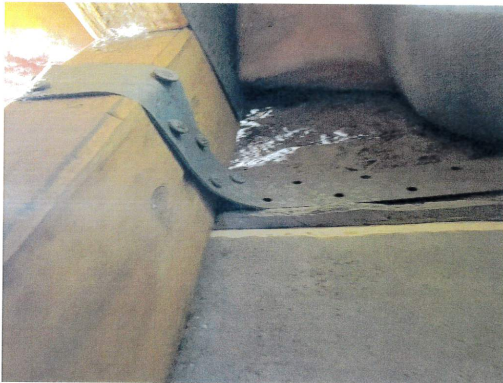
Figure 6 - Roof to Wall Attachment
