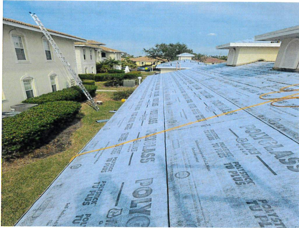
Figure 7 – Secondary Water Resistance
