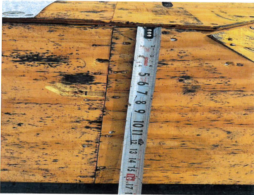
Figure 3 – Sheathing Fastener Spacing
