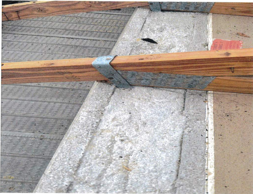
Figure 5 – Roof to Wall Attachment
