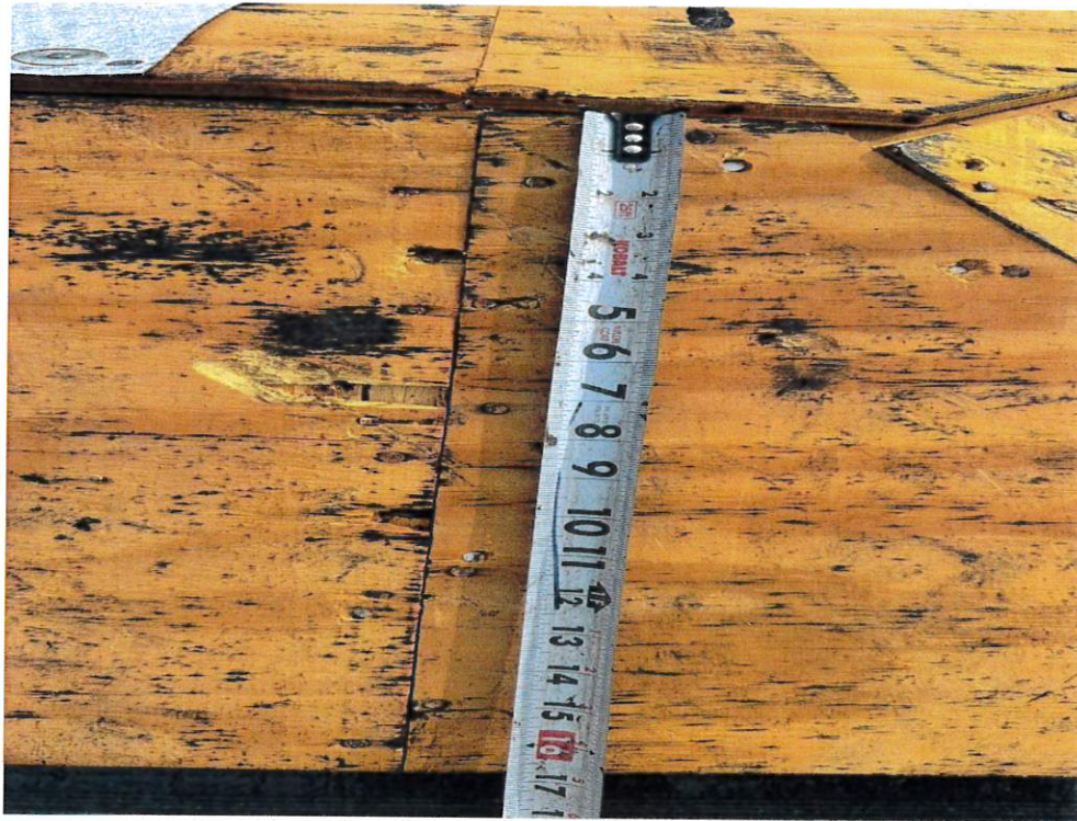
Figure 3 – Sheathing Fastener Spacing
