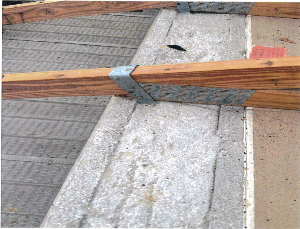
Figure 5 – Roof to Wall Attachment
