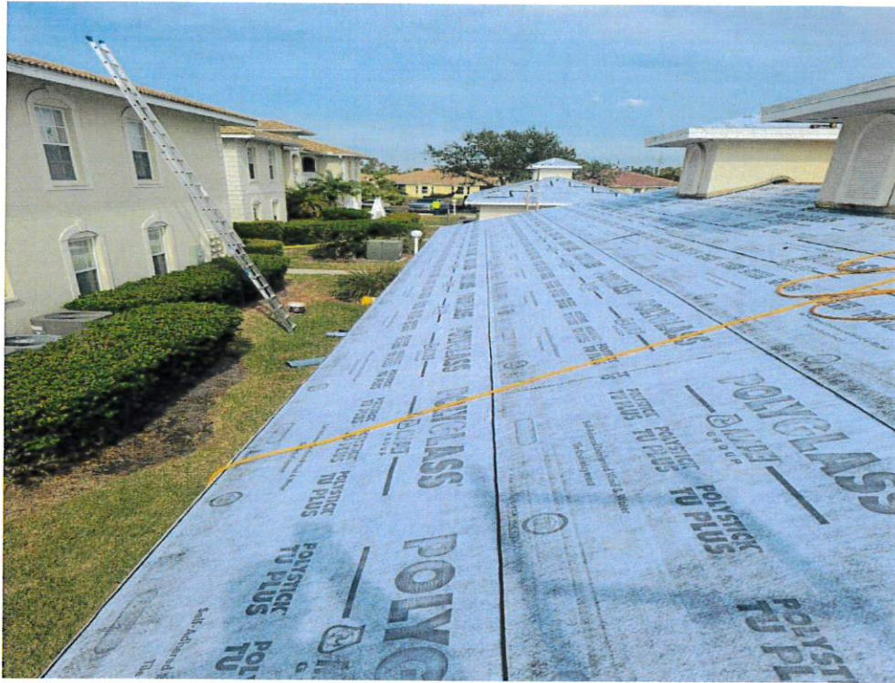
Figure 7 – Secondary Water Resistance
