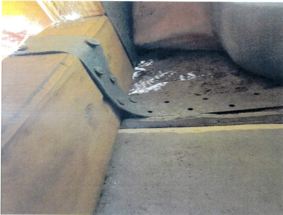
Figure 6 - Roof to Wall Attachment
