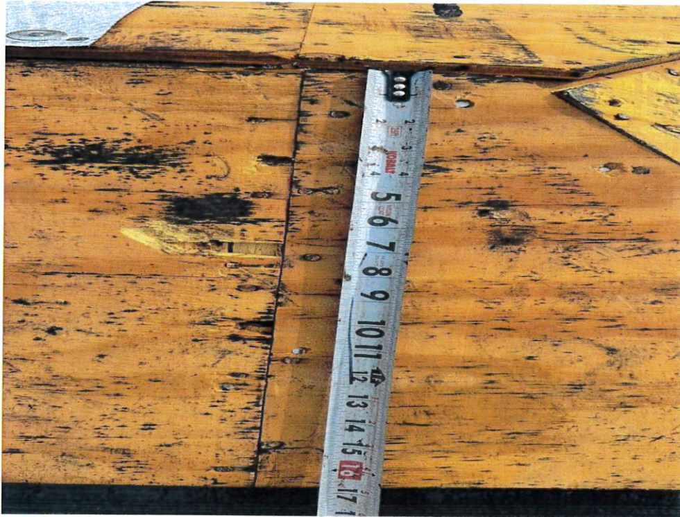
Figure 3 – Sheathing Fastener Spacing
