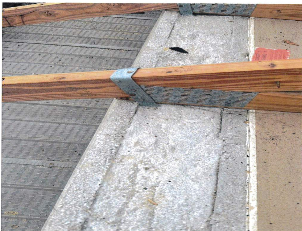
Figure 5 – Roof to Wall Attachment
