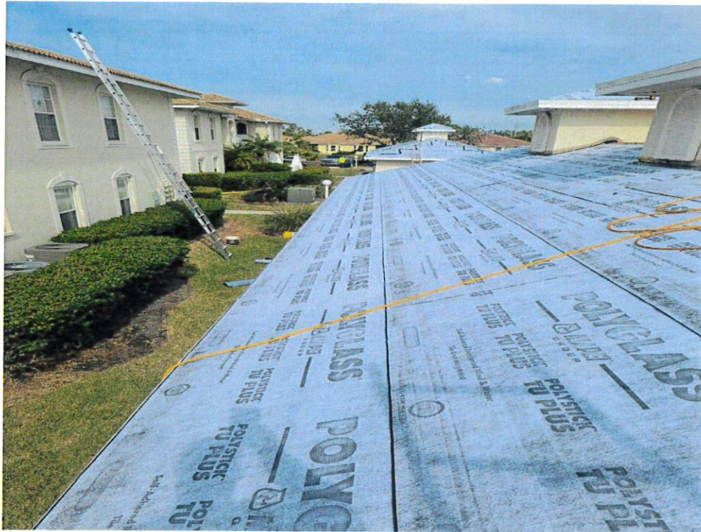
Figure 7 – Secondary Water Resistance
