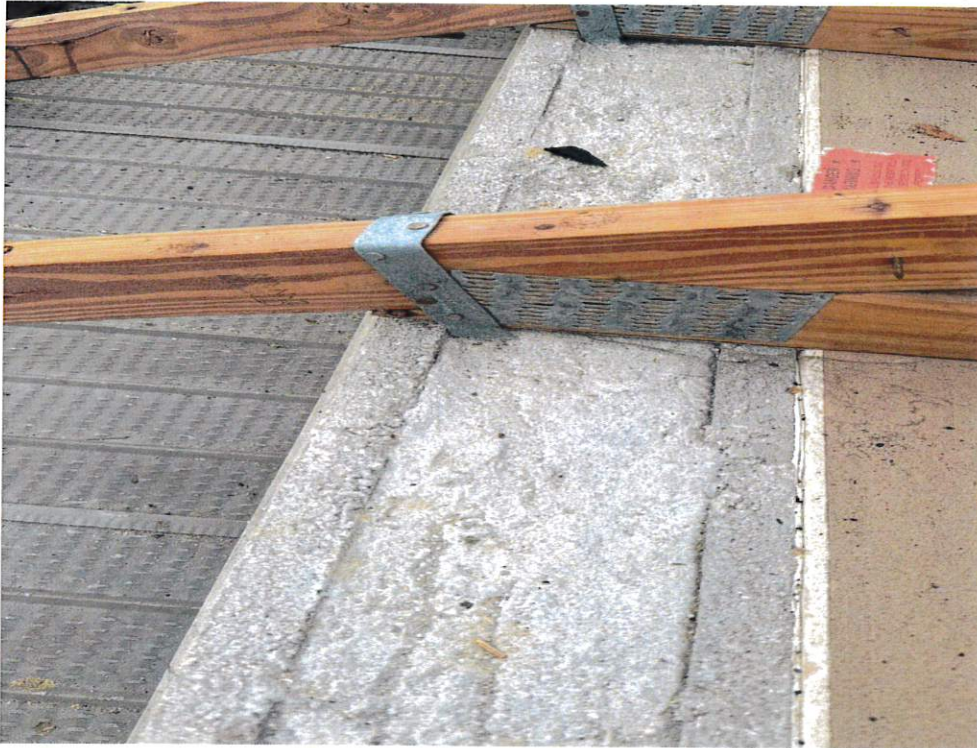
Figure 5 – Roof to Wall Attachment
