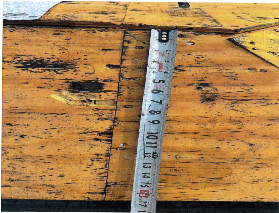
Figure 3 – Sheathing Fastener Spacing
