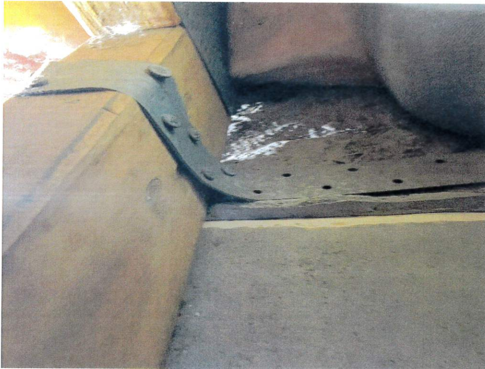
Figure 6 - Roof to Wall Attachment
