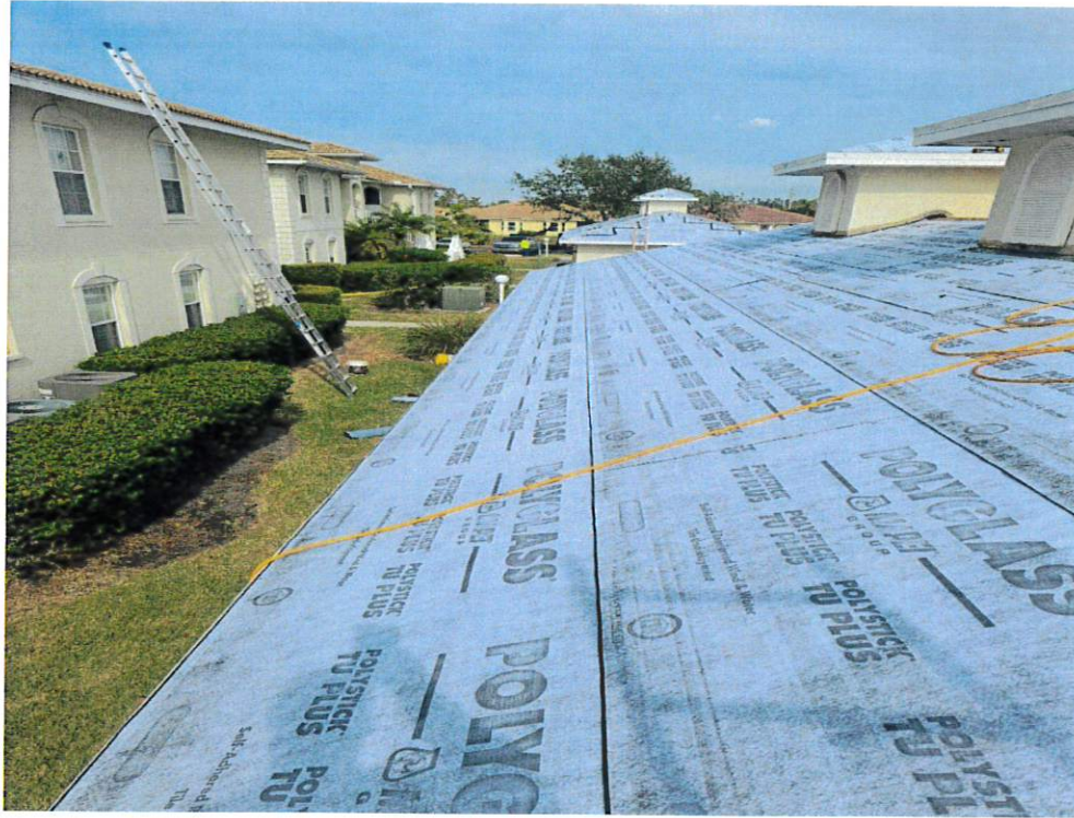
Figure 7 – Secondary Water Resistance
