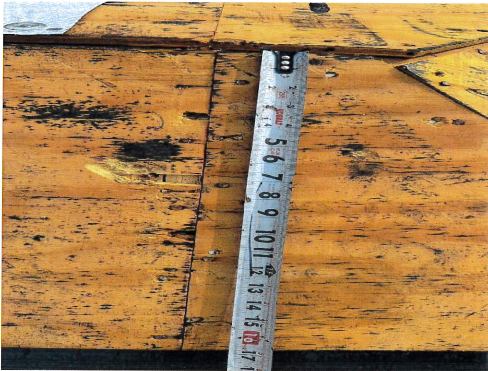
Figure 3 – Sheathing Fastener Spacing
