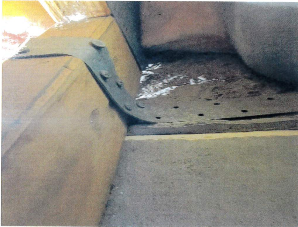
Figure 6 - Roof to Wall Attachment
