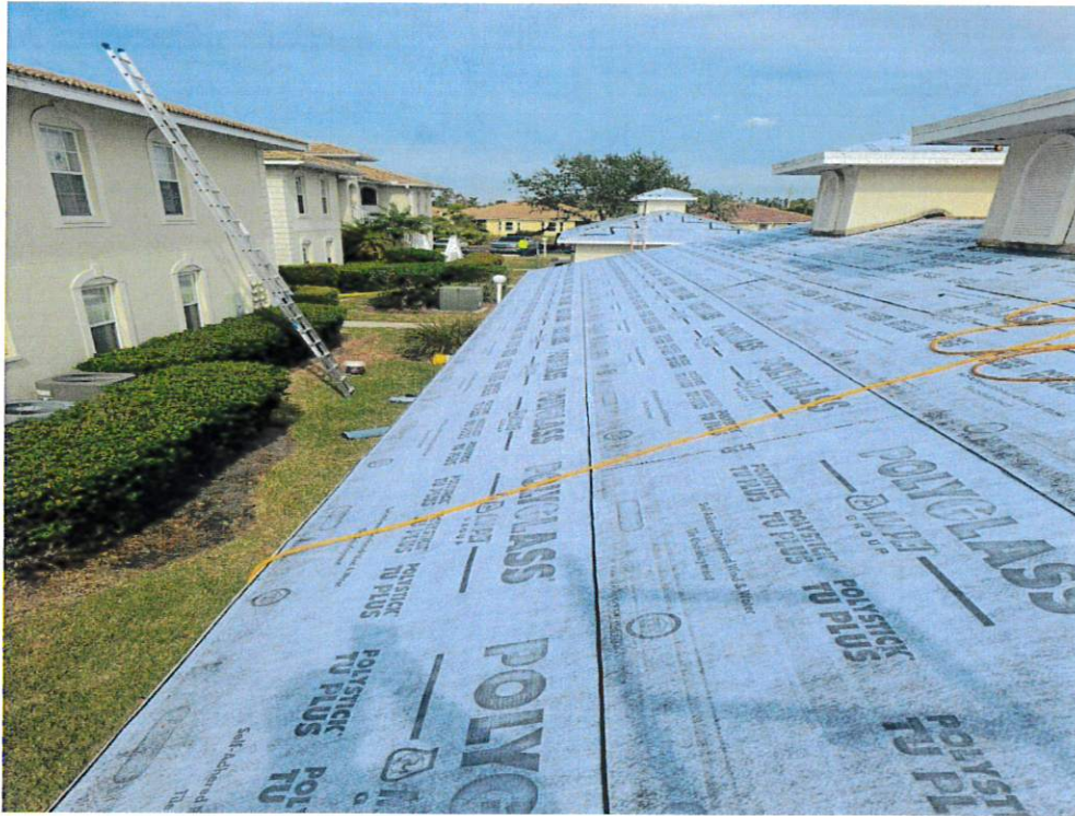
Figure 7 – Secondary Water Resistance
