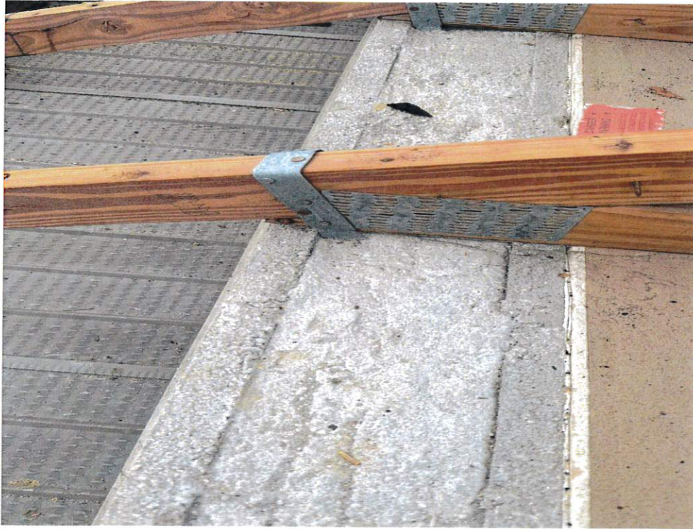
Figure 5 – Roof to Wall Attachment
